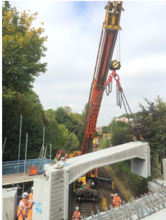
Figure 5 MVL3/34 Granville Street - Example of rail crane lifting bridge superstructure into position
