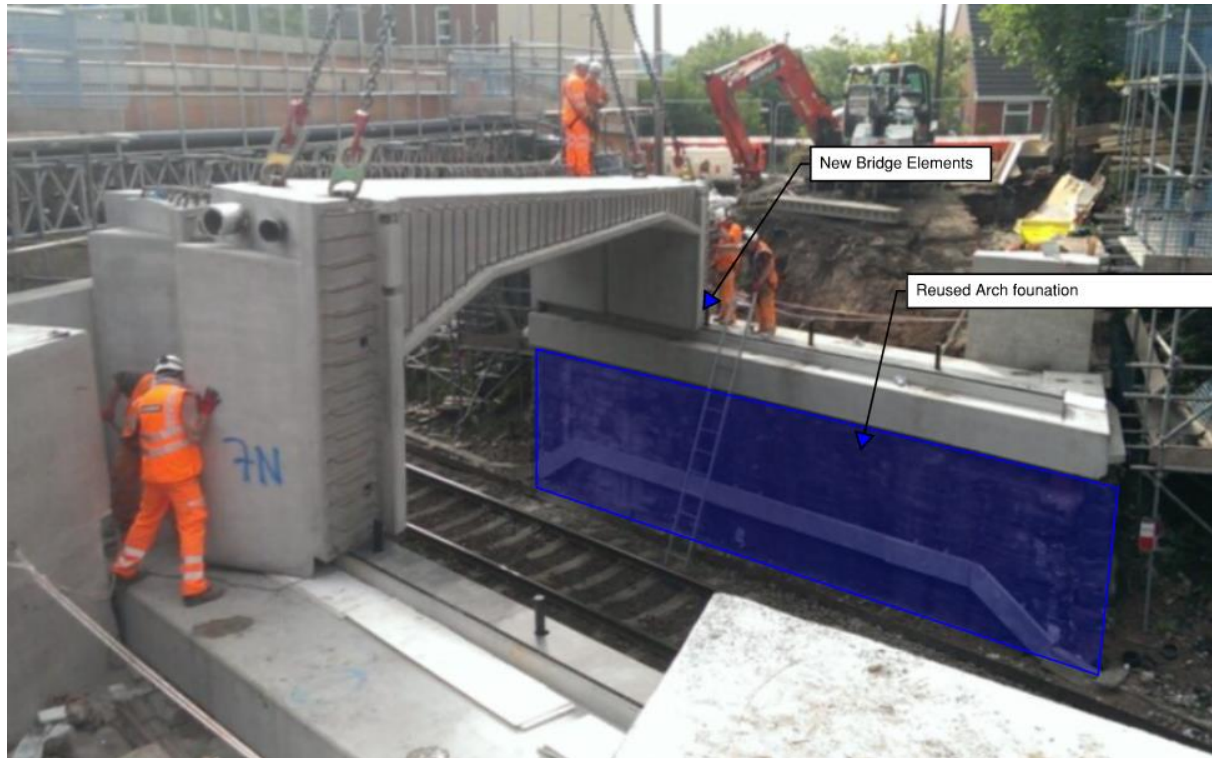
Figure 4 MVL1/34 Granville Street - Example of the reuse of an existing arch abutment
