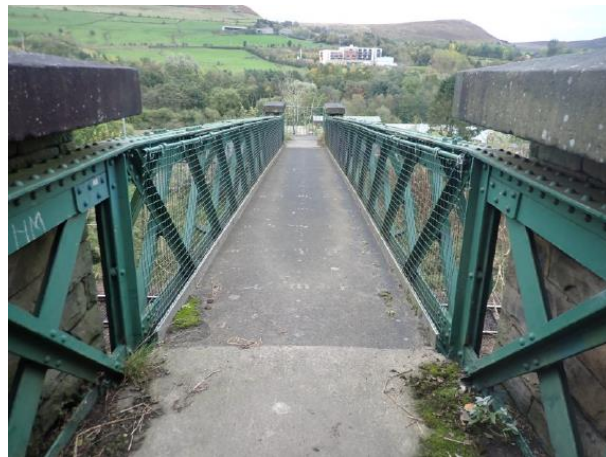
Figure 23 MVL3/18 View from highway level
