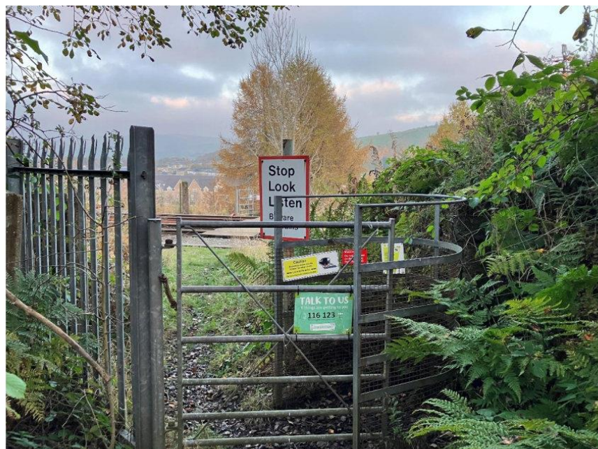
Down side approach
