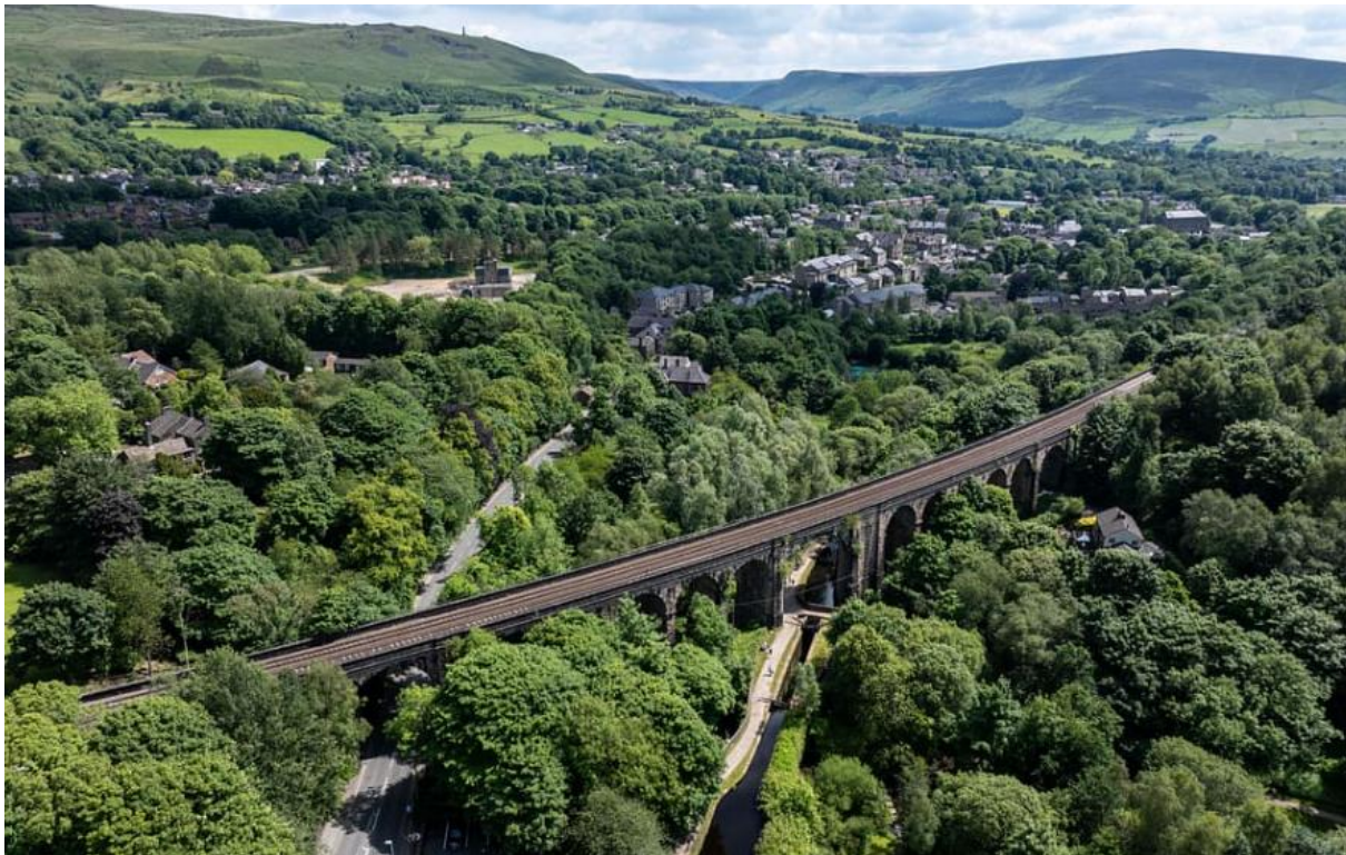
Figure 44 Areal View of MVL3/31
