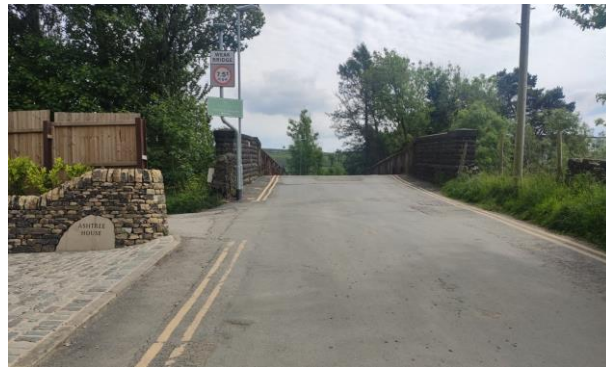
Figure 49 MVL3/36 View from highway level
