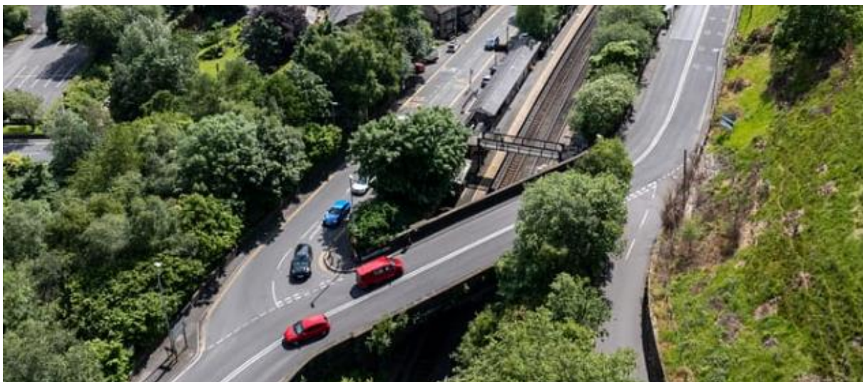
Figure 37 Areal view of MVL3/28 and Existing Station footbridge
