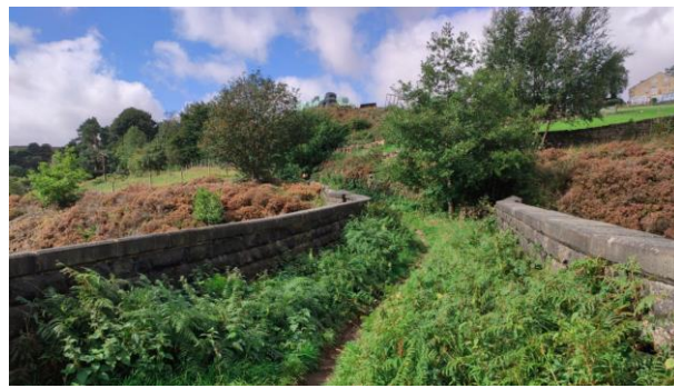
Figure 26 MVL3/20 View from highway level
