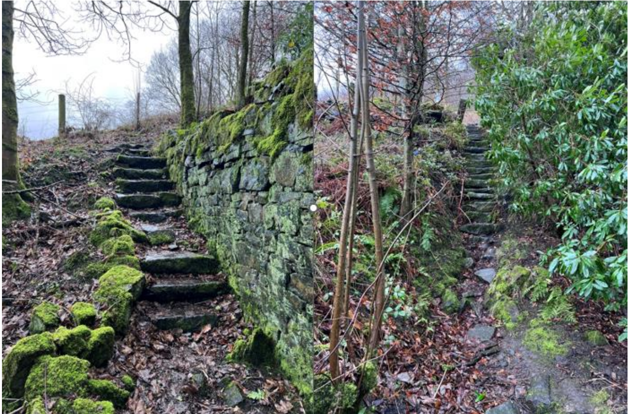
Figure 83 Stairs near intersection with Ladcastle Road
