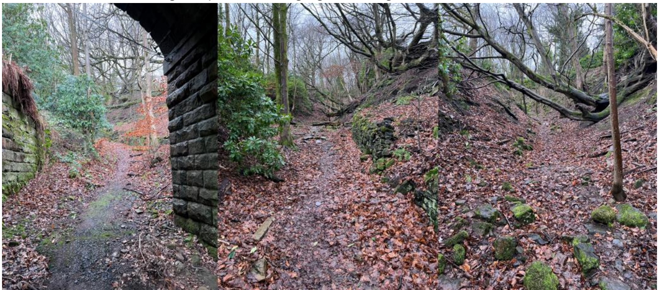
Figure 82 244SADD Between MVL3/29 and first set of stairs
