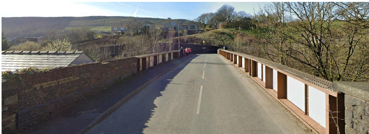
Figure 52 MVL3/39 View from Highway
