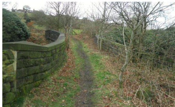
Figure 29 MVL3/23 View from highway level
