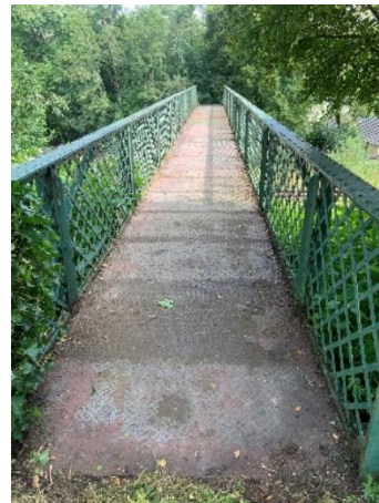
Figure 17 MVL3/10a View from footway level
