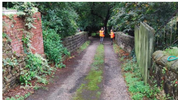
Figure 12 MVL3/7 View from highway level
