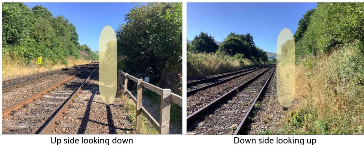
Figure 73 Moorgate Halt level crossing views
