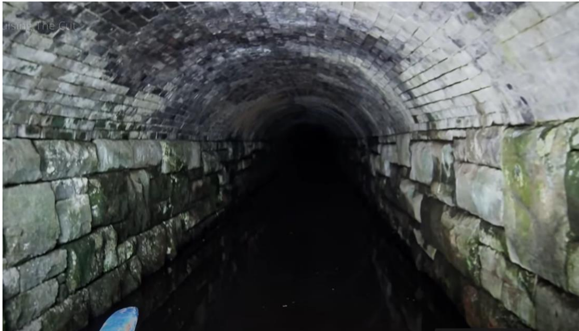
Figure 54 View of Standedge canal tunnel near to western portal
