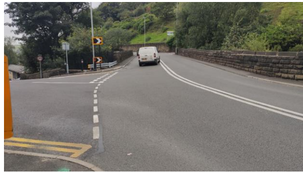
Figure 36 MVL3/28 View from highway level
