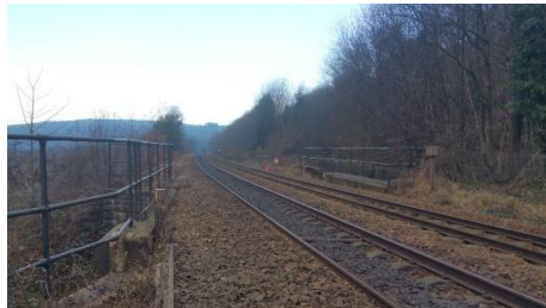
Figure 34 MVL3/25 View from track level
