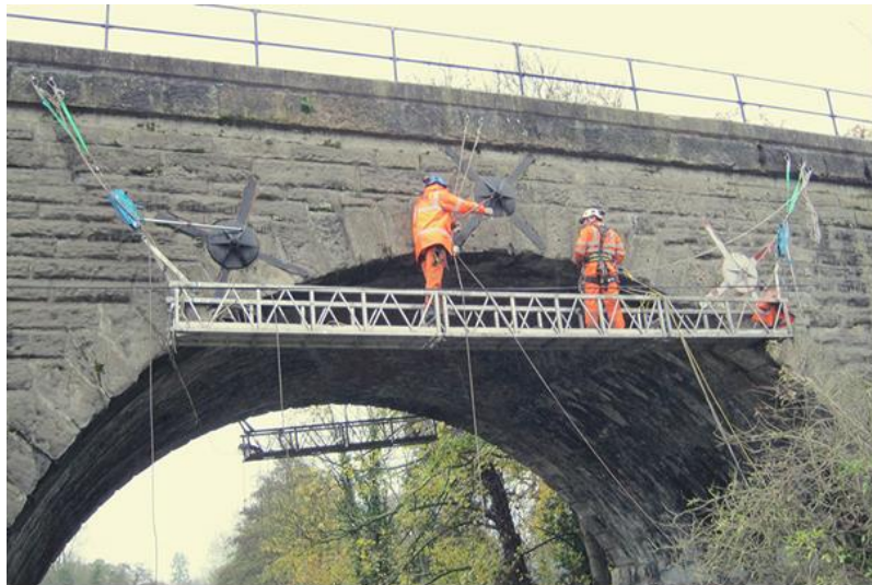
Figure 47 Indicative working platform during construction
