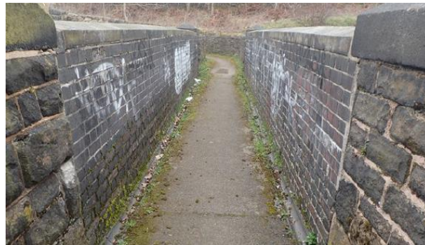
Figure 15 MVL3/8 View from footway level
