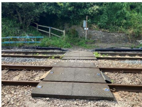
Up side across crossing
