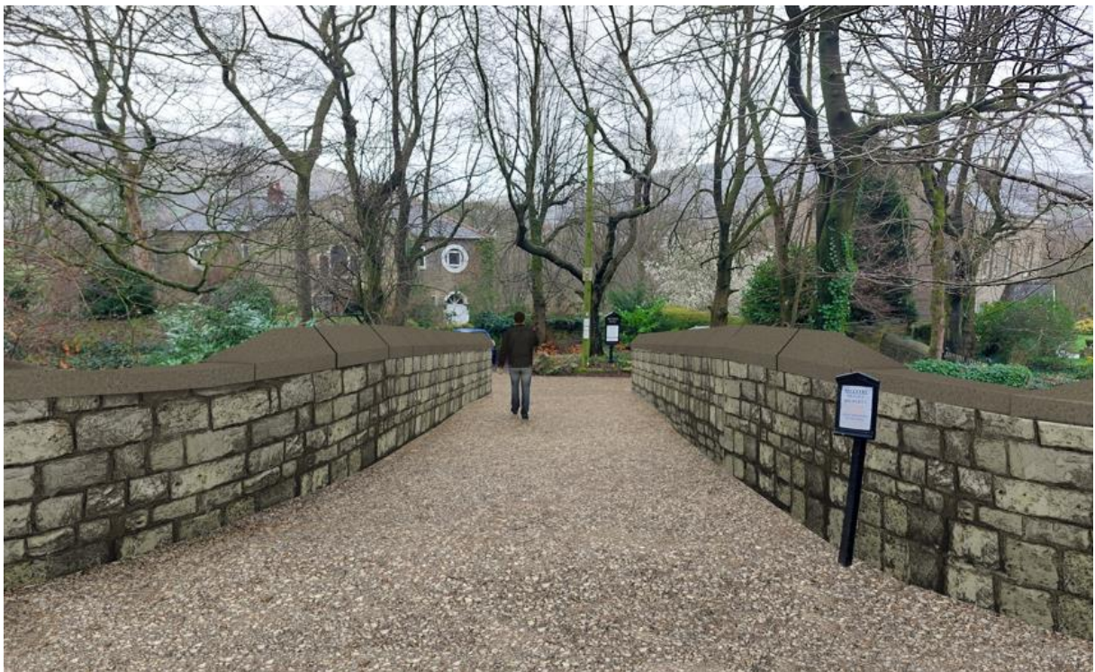
Figure 13 - Reconstructed MVL3/7 viewed from highway level
