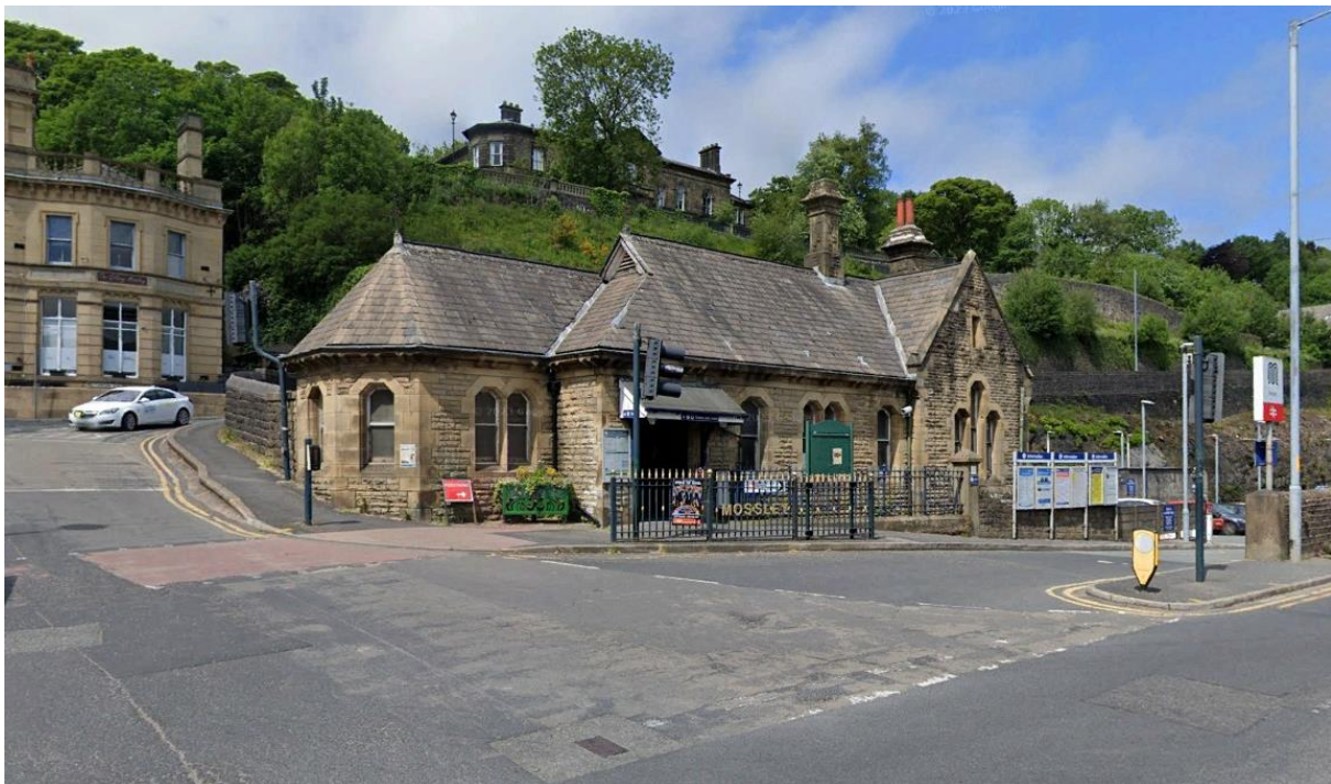
Figure 59 View of Station building from Manchester Road
