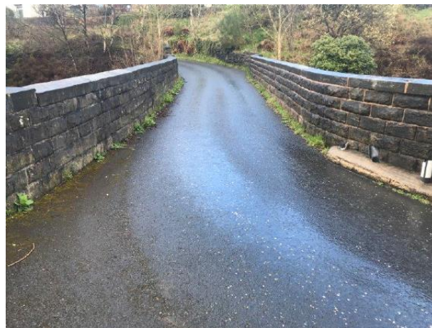
Figure 20 MVL3/17 View from highway level
