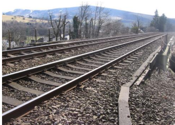
Figure 43 MVL3/29 View from track level
