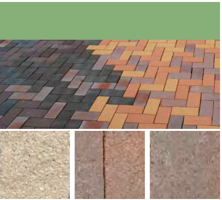
Permeable concrete block mix to cycle parking
