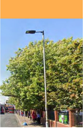
Column lighting to Highway authority standards
