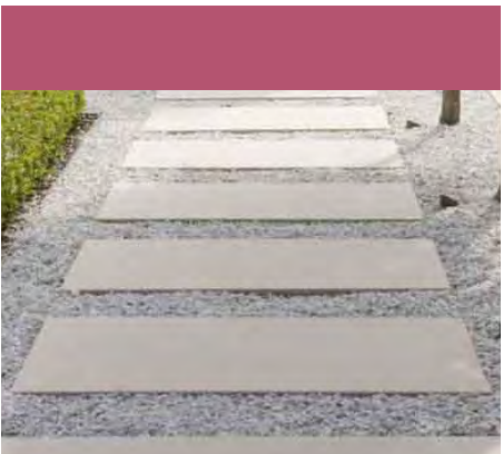
Concrete stepping stones & gravel to paths for private residential amenity terraces
