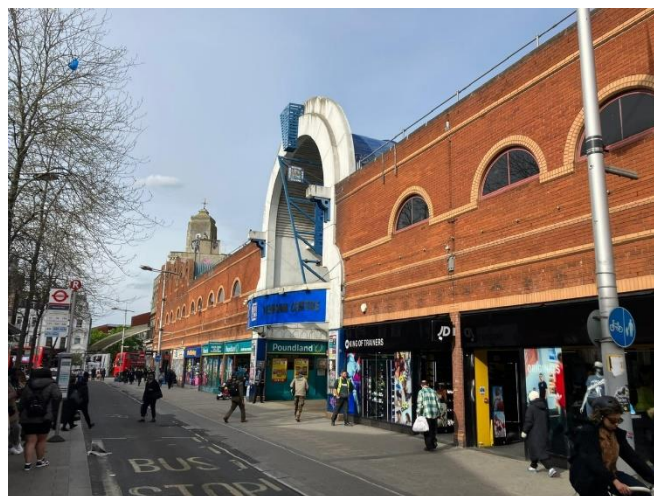
Retail Units fronting Rye Lane
