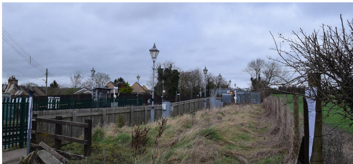
Figure 21: View from the former eastern gate of Tackley Level Crossing, showing the station and bridge site from the level crossing to the south. (S. Khalifeh/Taziker, 2024).
