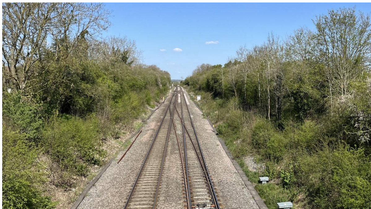
Figure17: View from the existing temporary footbridge, looking north.
