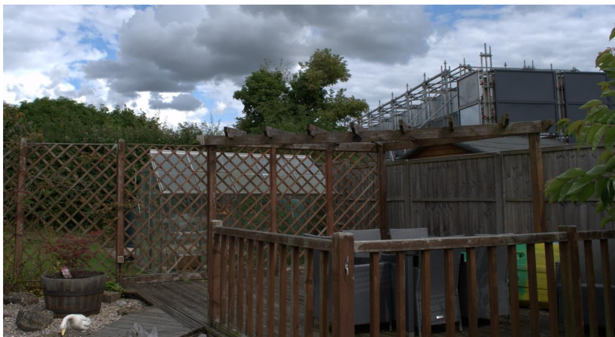
Figure 25: View from the back garden of 59 Nethercote Road. The toe of the new staircases would be behind the fence roughly in line with the top of the temporary stairs when viewed from this angle.
