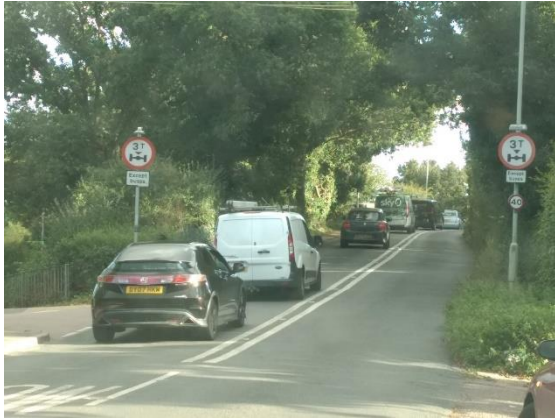
Station road - Smallford Lane bridge
