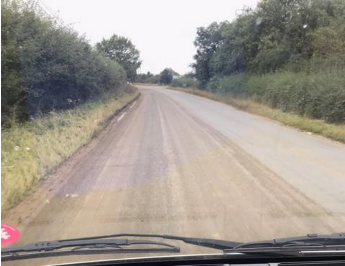
Mud on Coursers Road between site exit and Bell roundabout photo taken 8 th October 2021 at 9.42am.
