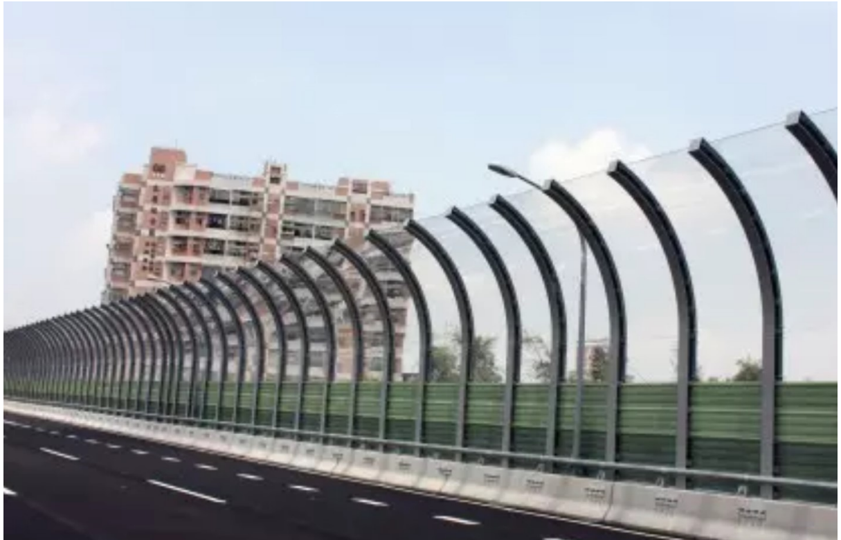
Figure 5.2: Example of Cantilevered Acoustic Barrier (Picture of the Expressway Section near the Tzu Chi Hospital at Taichung, Taiwan, photo courtesy of Raychung Acrylic)
