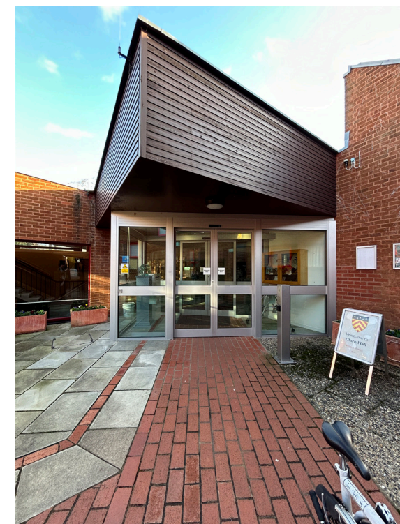
New entrance lobby
