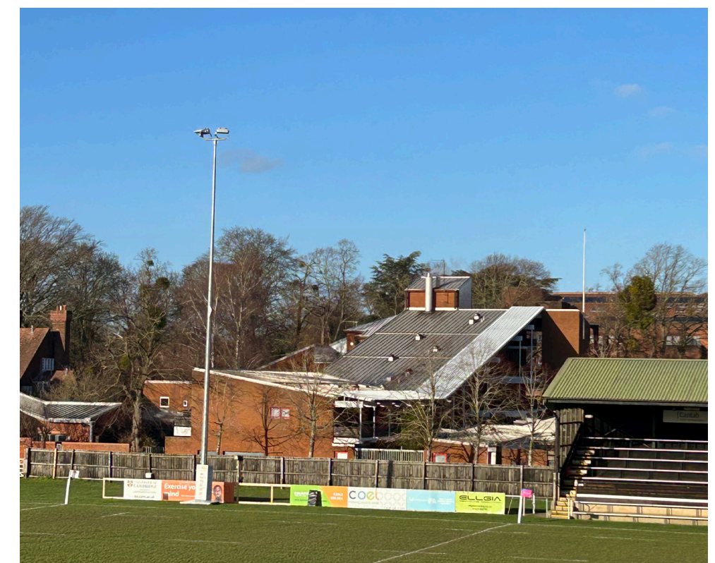
View from the Rugby Ground looking north showing south facing roof surface which could accommodate pv/solar thermal panels
