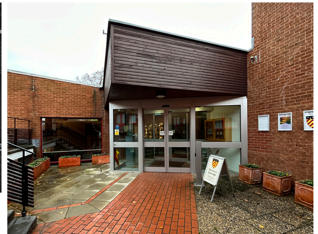
New entrance draft lobby
