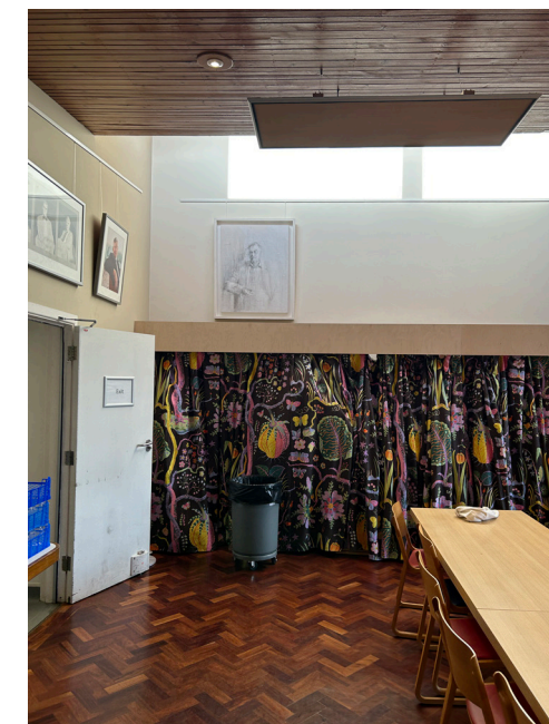
Curtains and suspended panels added to improve acoustics in the dining hall.
