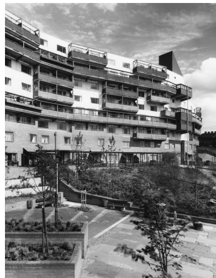
Byker Wall, Newcastle-upon-Tyne
