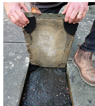
Asphalt covering beneath paving
