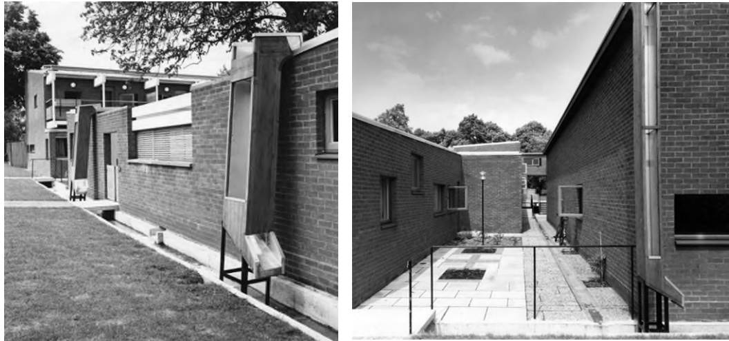
Figure 19 Original photos taken in 1970 of connecting paths, channel, rainwater chutes and bridges
