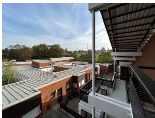
Figure 13 View looking south across roof tops
