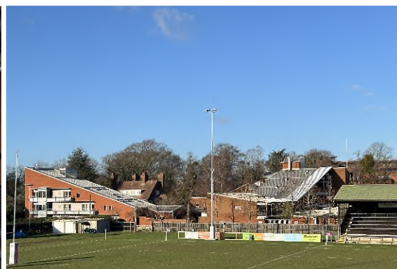
Figure 14 View from Rugby ground towards Clare Hall
