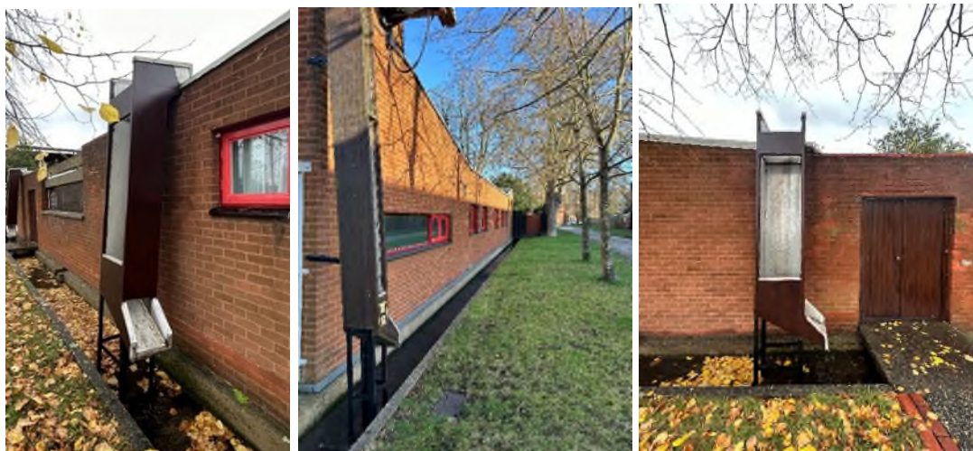
Figure 23, 24 and 25 Waterspouts and water channel along South boundary.
