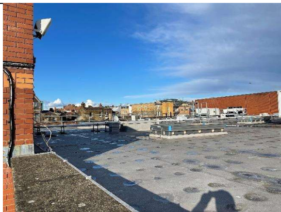
Photograph 27: Roof of the Aylesham Centre/Morrisons.
