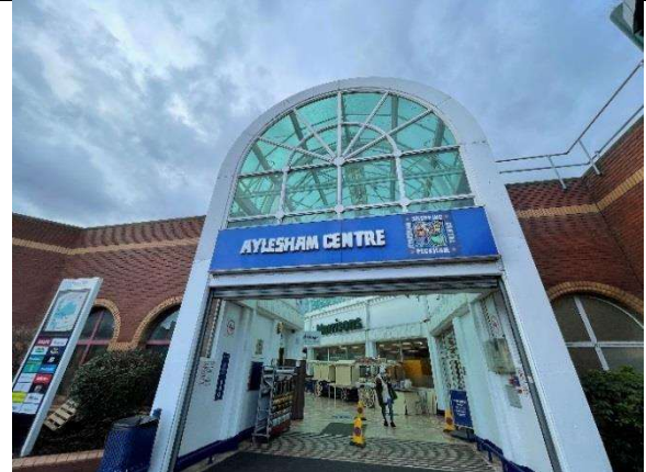
Photograph 20: The east façade of the building
