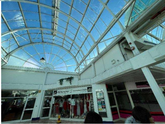
Photograph 5: Glass atrium within Aylesham Centre
