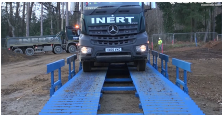
Figure 9: Dry Wheel Wash Station in use
