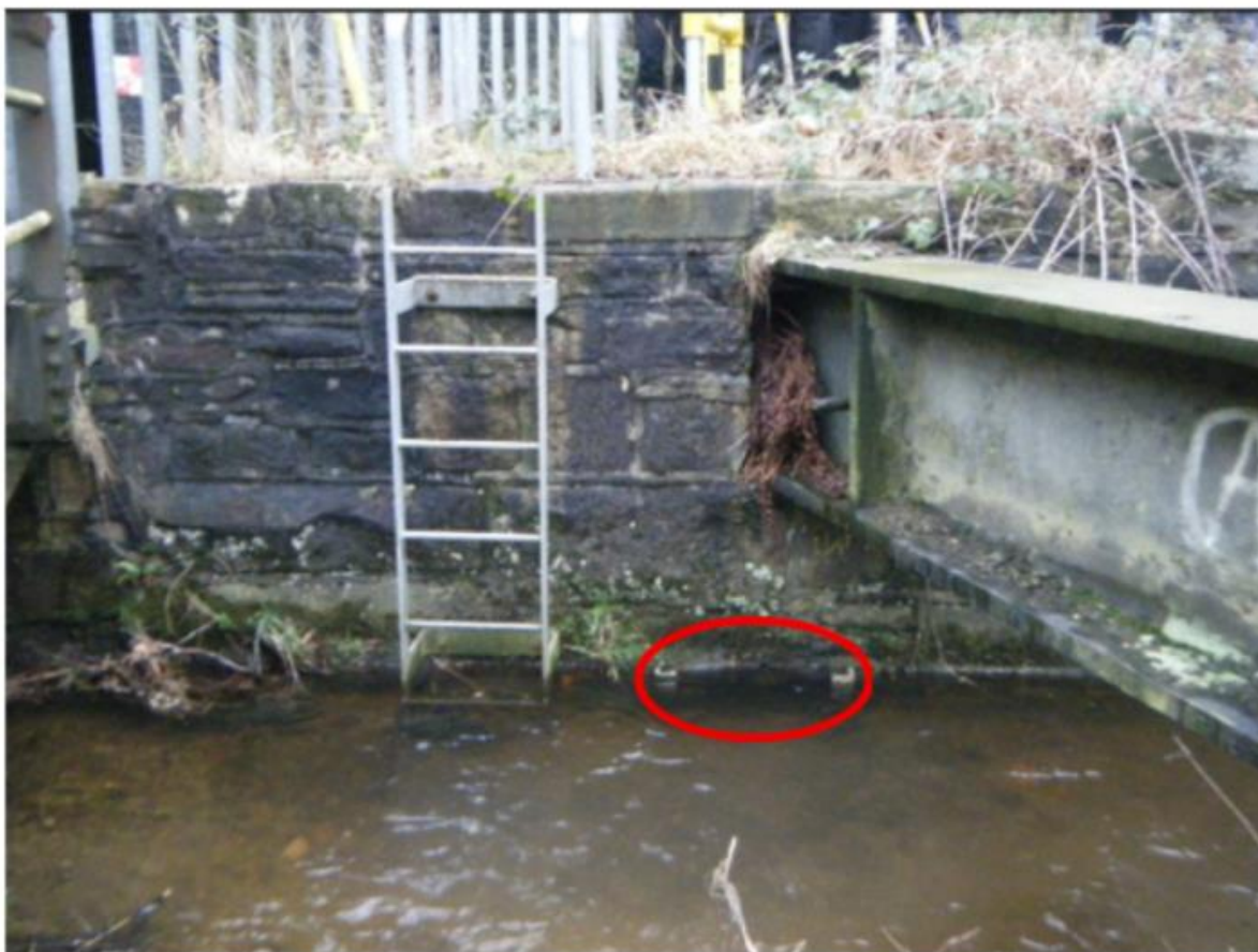
Fig. 3 - Brunclough abstraction orifice
