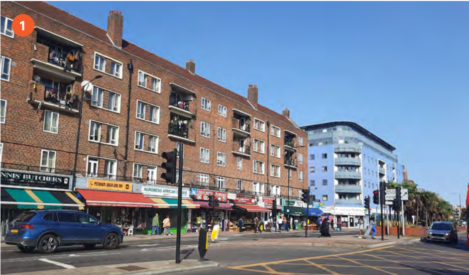
Peckham High Street Peckham High Street is a busy thoroughfare upon which the volume of traffic compromises the retail experience and public realm. The road serves a number of bus routes and has large volumes of traffic as it provides a strategic link to Central London. It consists largely of independent stores.
