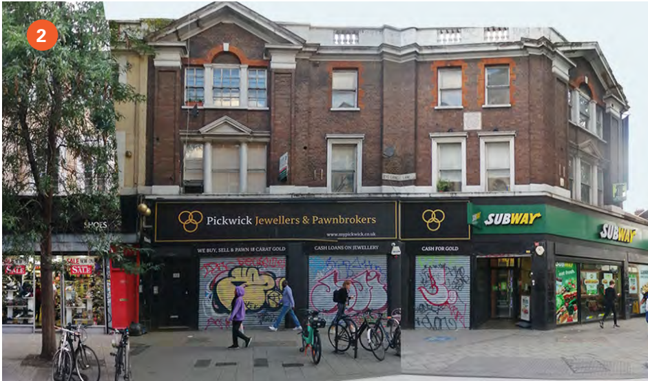
Rye Lane north-west This character area is one of the busiest sections of Rye Lane in terms of pedestrian traffic, cyclists and buses. It comprises of a combination of chain and independent stores located within historically residential properties that have been converted to mixed-use buildings.
