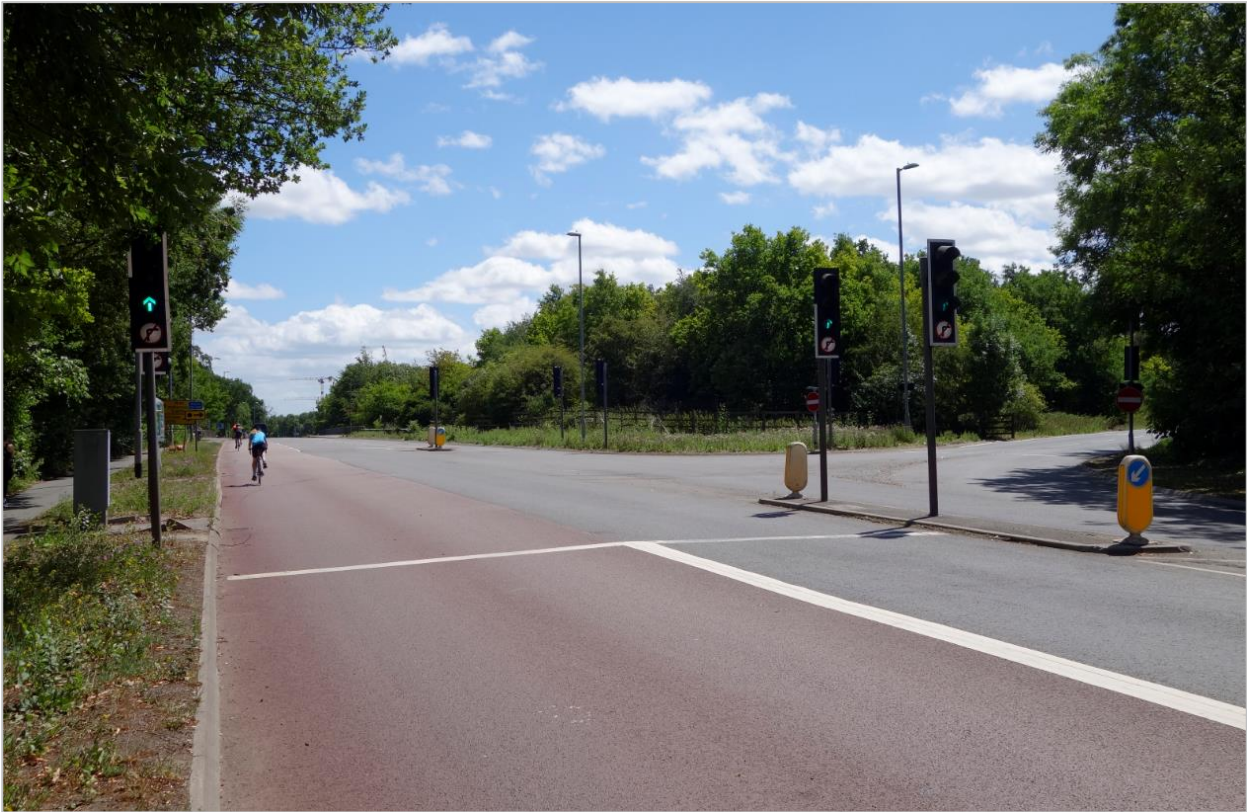
Figure 18: Current M11 exit junction with Madingley Rd (© 2020 Edward Leigh)
