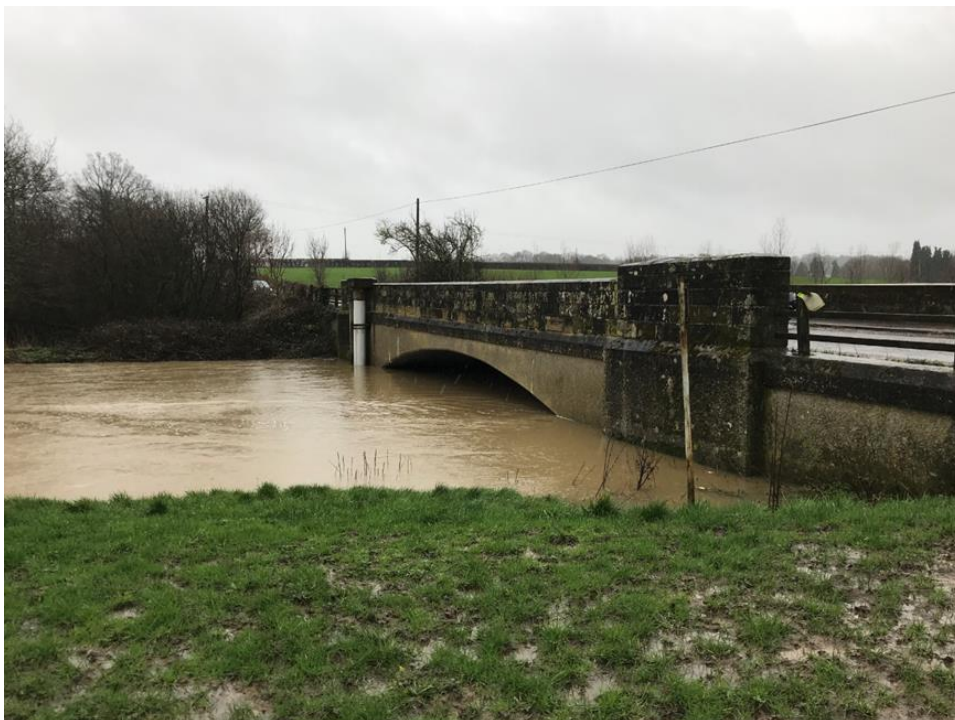
Figure 6: The bridge on Ensfield Road over the River Medway, 12:37 on 16 February 2020
