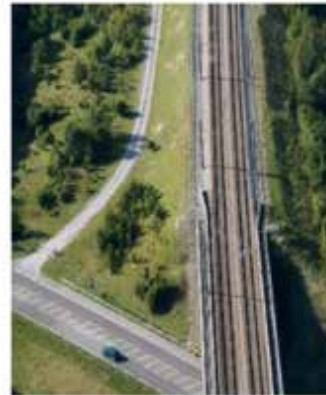
Maintenance Access Track
