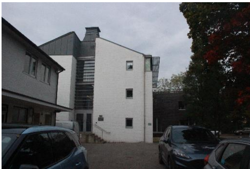
Above: View of Salje Building accommodation south elevation Image Capture: October 2025
