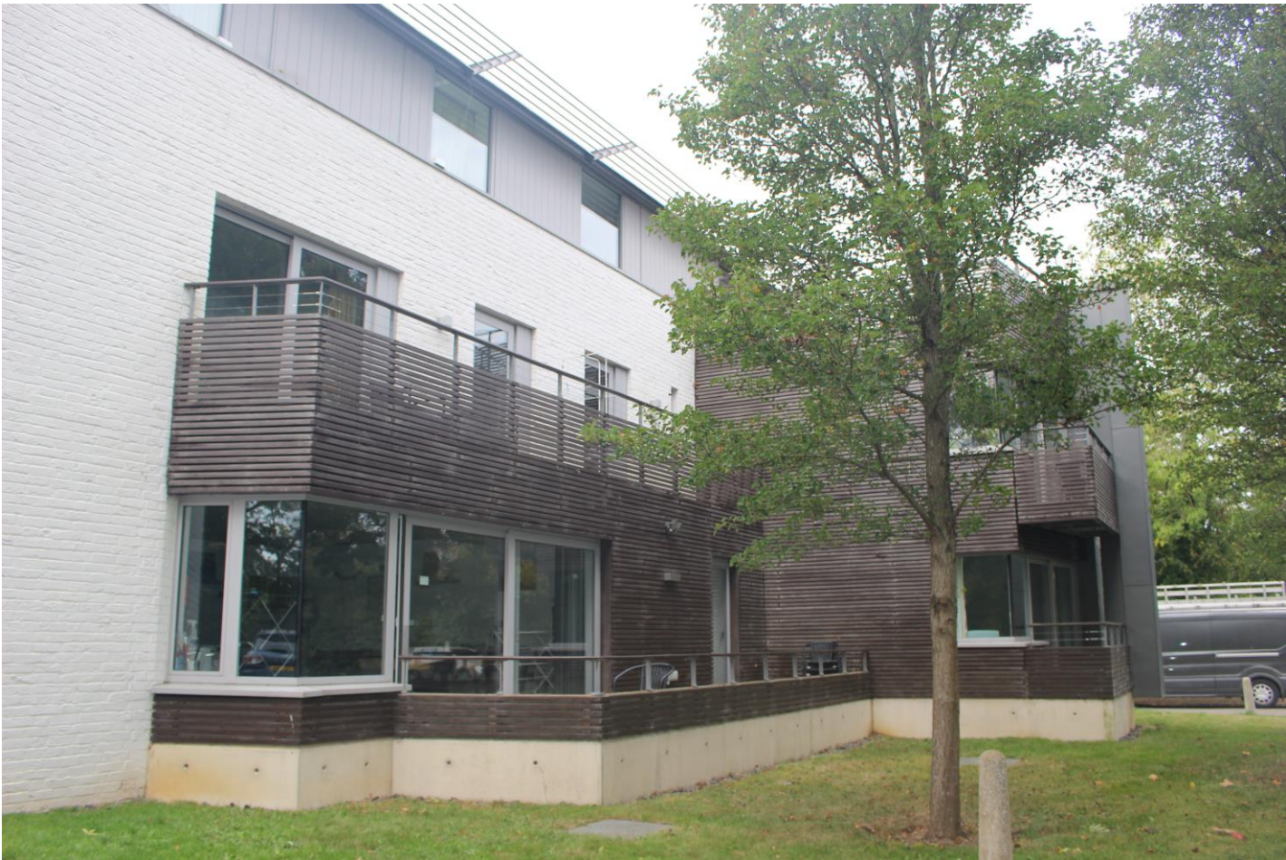
Above: Salje Building east elevation
