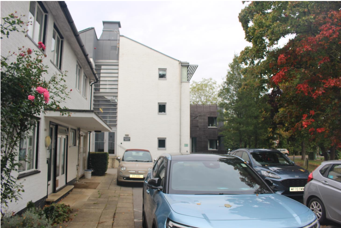
Above: Salje Building south elevation
