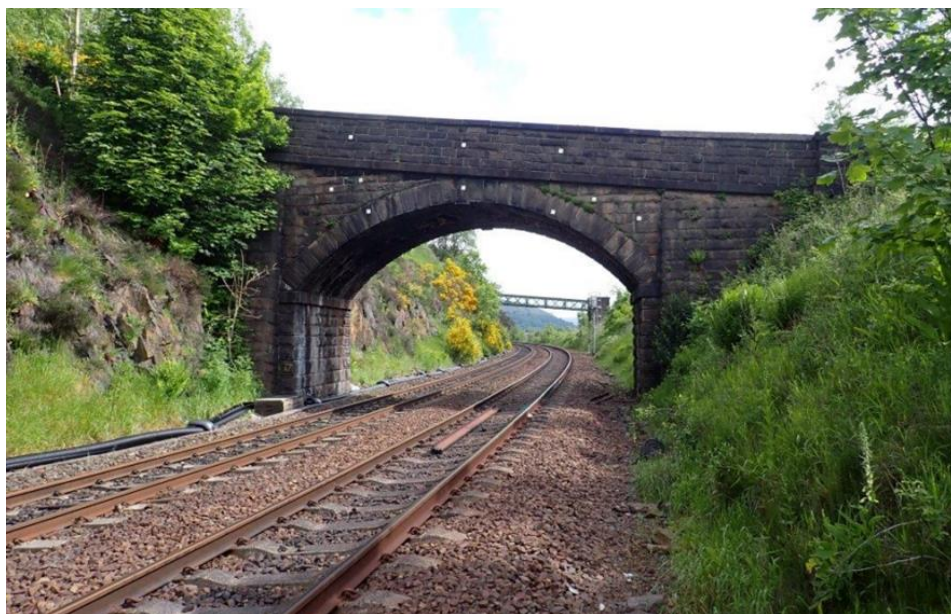
Insert 5-8 Roughtown Road Overbridge (MVL3/17), south-east elevation.
