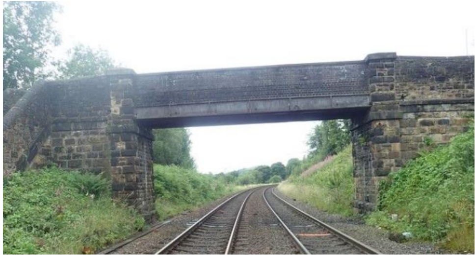
Insert 5-3 Springbank Lane Footbridge (MVL3/8) northern elevation
