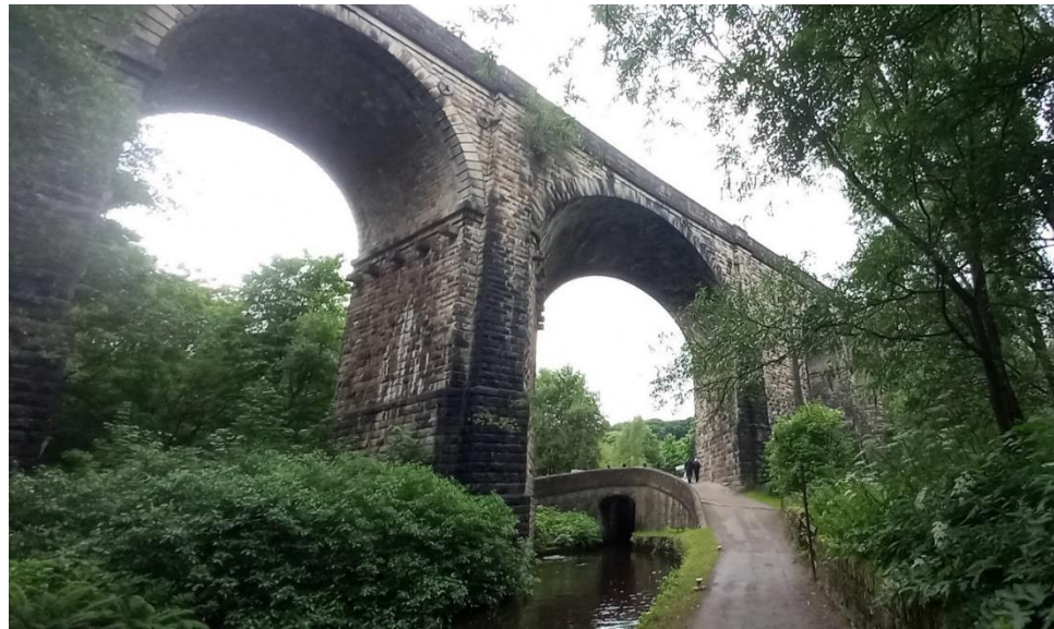
Insert 5-12 Uppermill Viaduct (MVL3/31) and tail bridge No.75 (NHLE 1356719) on the Huddersfield Narrow Canal showing their close relationship and use of skew arch.
