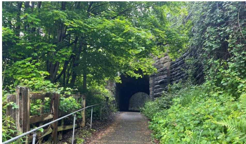
Insert 5-2 Shaw Hall Bank Road Footway (MVL3/26), south elevation.
