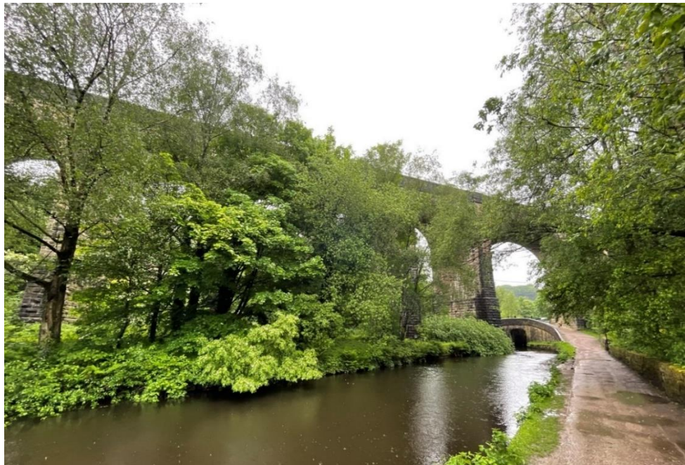
Insert 5-5 Uppermill Viaduct (MVL3/31) viewed from the canal from the south-east.
