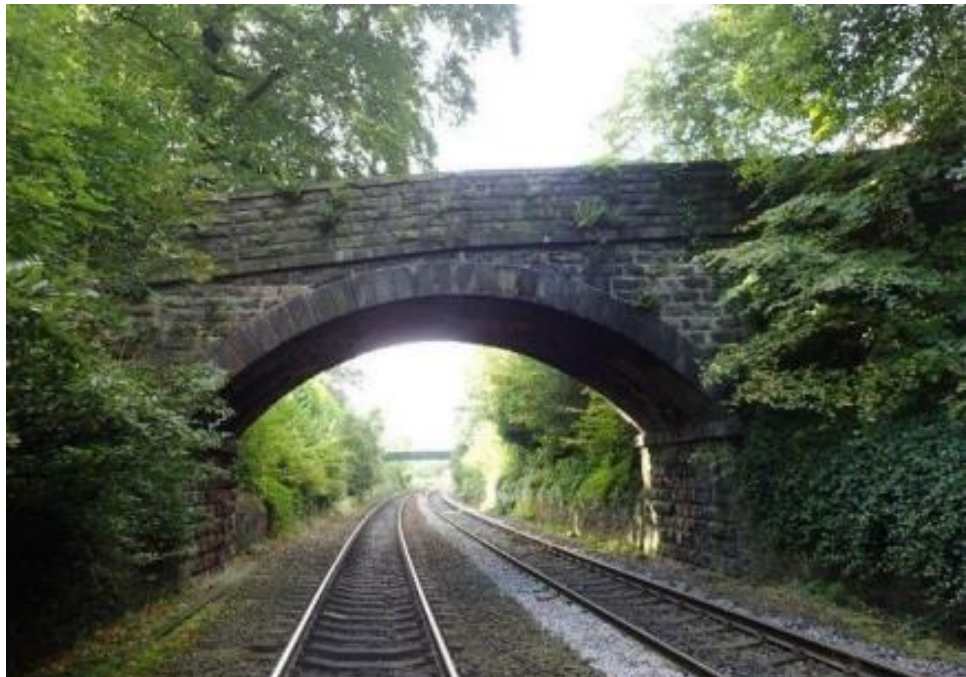
Insert 1-2 North-east elevation of Heyrod Hall Overbridge (MVL3/7).
