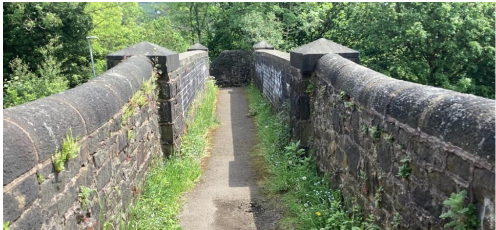
Insert 5-4 Springbank Lane Footbridge (MVL3/8) footpath and parapets atop of the bridge
