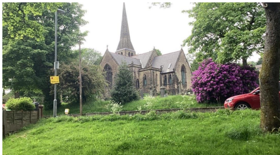
Insert 5-5 View of Christ Church from south of Church Road
