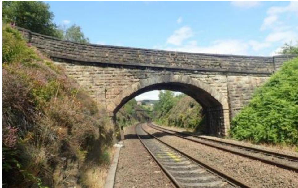
Insert 5-8 Wright's Mill Overbridge (MVL3/20), south elevation (Network Rail, 2022).
