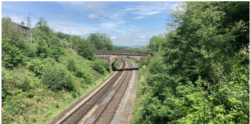
Insert 5-8 View north from Springbank Lane Footbridge (MVL3/8) to Spring Bank Lane Overbridge (MVL3/9).
