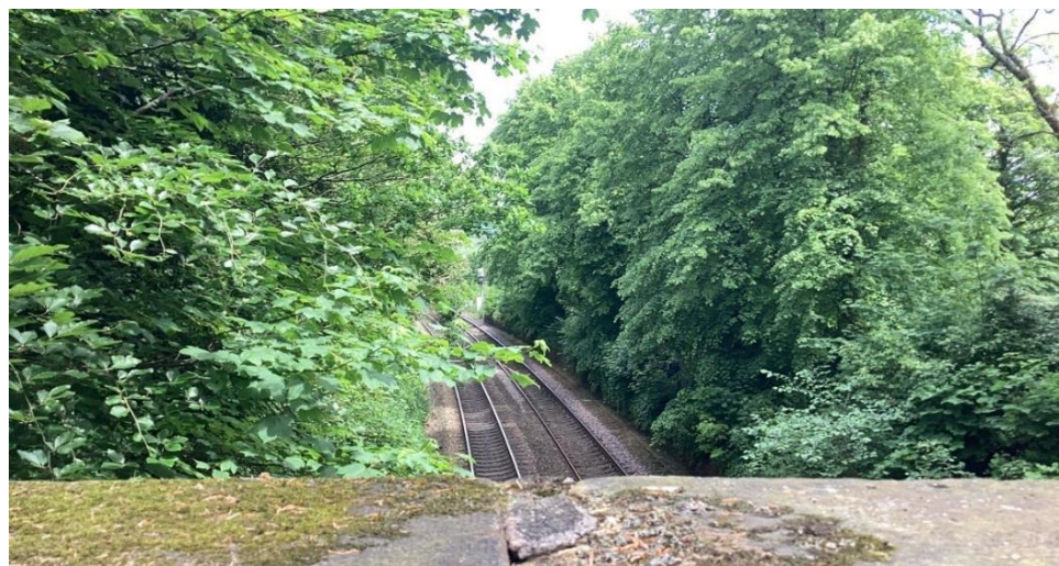
Insert 5-6 Heyrod Hall Overbridge (MVL3/7), view across the bridge parapet looking south-west
