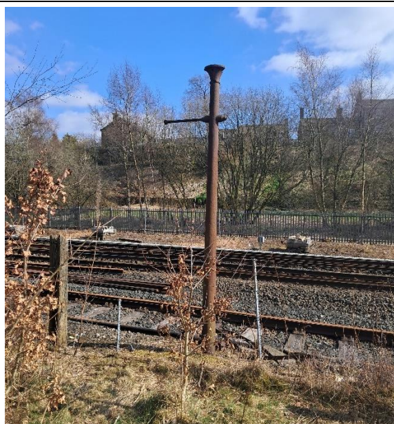
Cast iron gas lamp post located within Network Rail land boundary.
