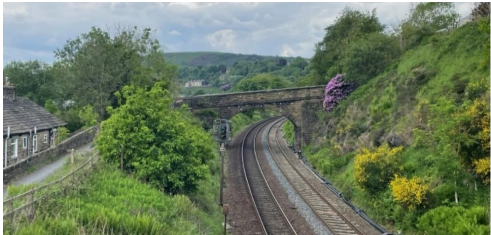
Insert 5-13 Roughtown Road Overbridge (MVL3/17), view looking south-west from the across the bridge deck.
