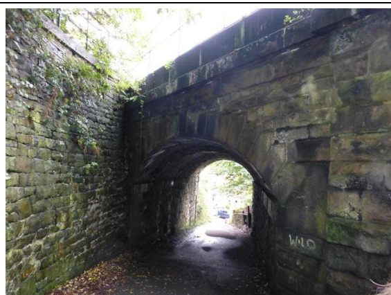
Railway accommodation underbridge MVL3/26, Footway © Historic England
