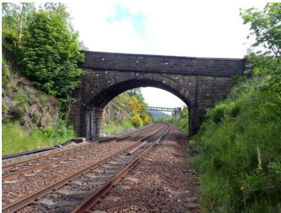
Insert 1-1 Roughtown Road Overbridge (MVL3/17), view from south.
