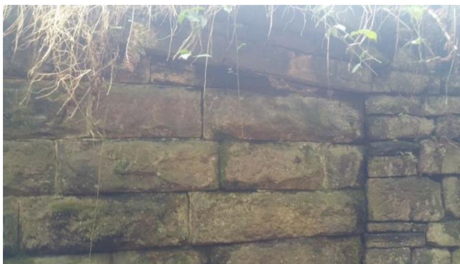
Insert 1-2 Shaw Hall Bank Road Footway (MVL3/26), soffit and masonry walling.
