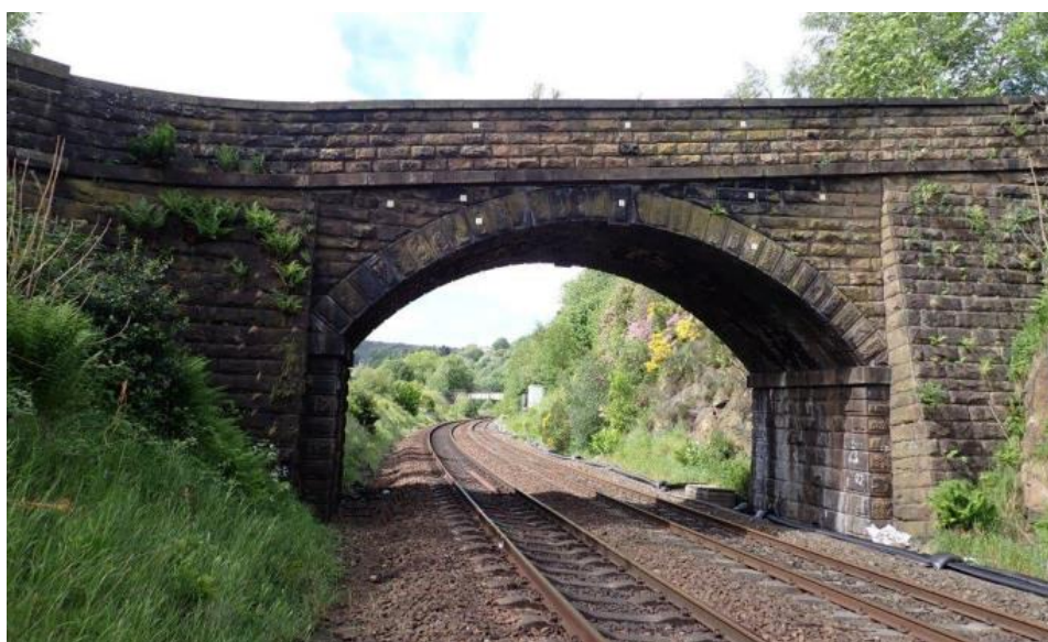
Insert 5-9 Roughtown Road Overbridge (MVL3/17), north-west elevation.
