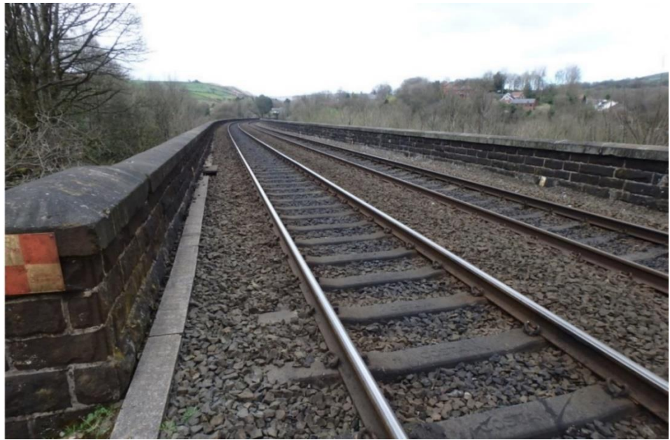
Insert 5-6 Deck of Uppermill Viaduct (MVL3/31), viewed from the southern end of the structure, showing parapets
