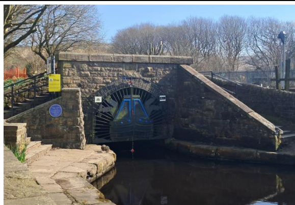
Entrance to Standedge Canal Tunnel (MVL3/39A). March 2025.
