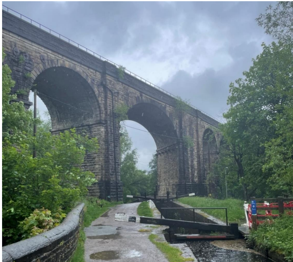
Insert 5-4 Uppermill Viaduct (MVL3/31) viewed from the canal to the north-west with Lock 23 of the Huddersfield Narrow Canal visible in the foreground.
