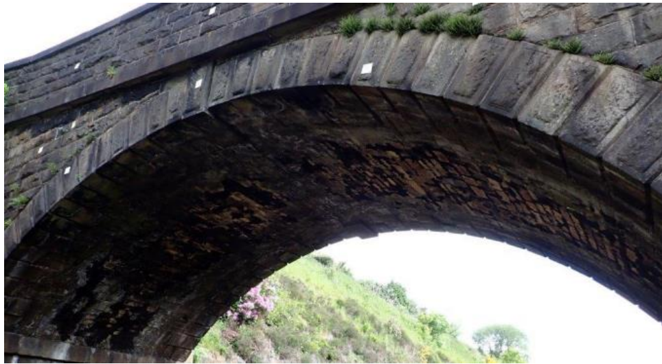
Insert 5-10 Roughtown Road Overbridge (MVL3/17), detail of arch and soffit
