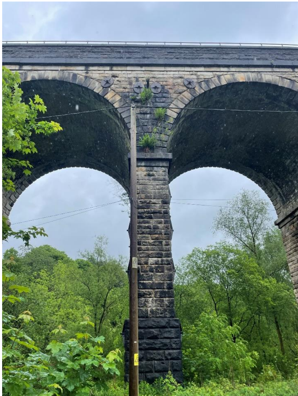
Insert 5-7 View of typical span detailing on the western elevation of the Uppermill Viaduct (MVL3/31)
