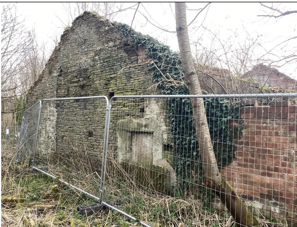
West gable elevation of the barn at Printworks Office Compound
