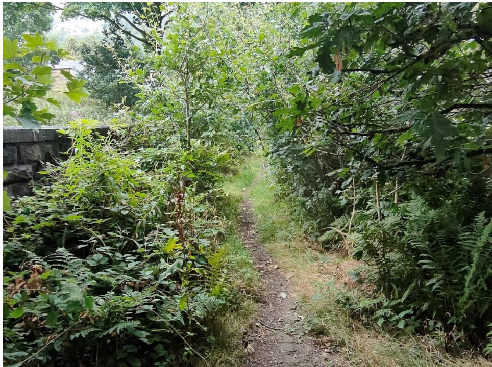
Insert 5-4 View south-west across the deck of Wright's Overbridge (MVL3/23).
