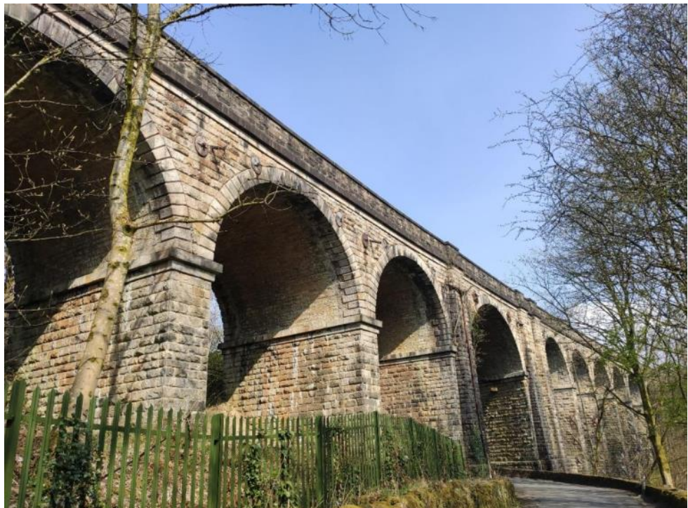
Insert 5-11 Uppermill Viaduct (MVL3/31), eastern elevation viewed from Den Lane.
