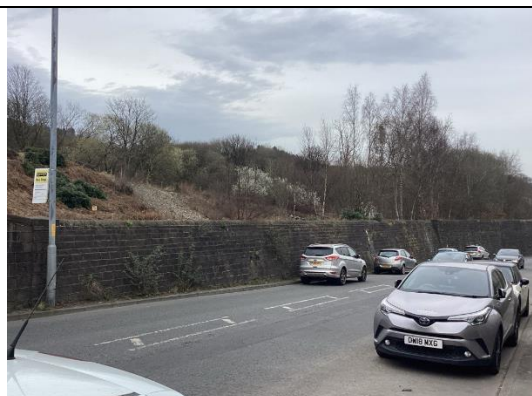
Retaining wall fronting Manchester Road, March 2025.
