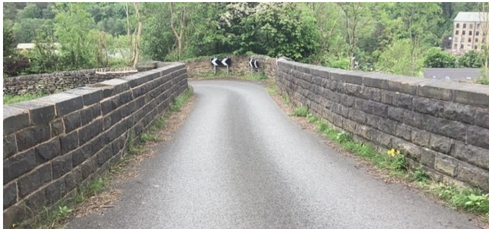
Insert 5-11 Roughtown Road Overbridge (MVL3/17), view east across the bridge deck
