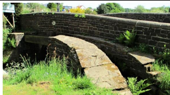
Huddersfield Narrow Canal No. 66 Bridge
