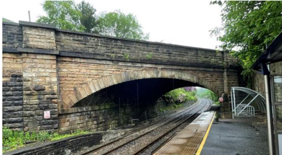
Insert 1-1 Oldham Road Underbridge (MVL3/28), south-western elevation
