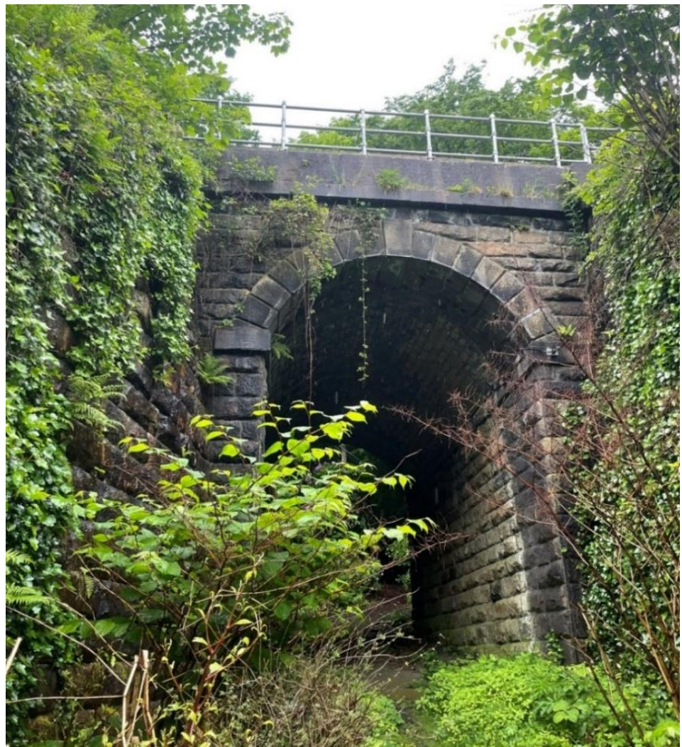
Insert 1-1 South elevation of Wickens Underbridge (MVL3/29)
