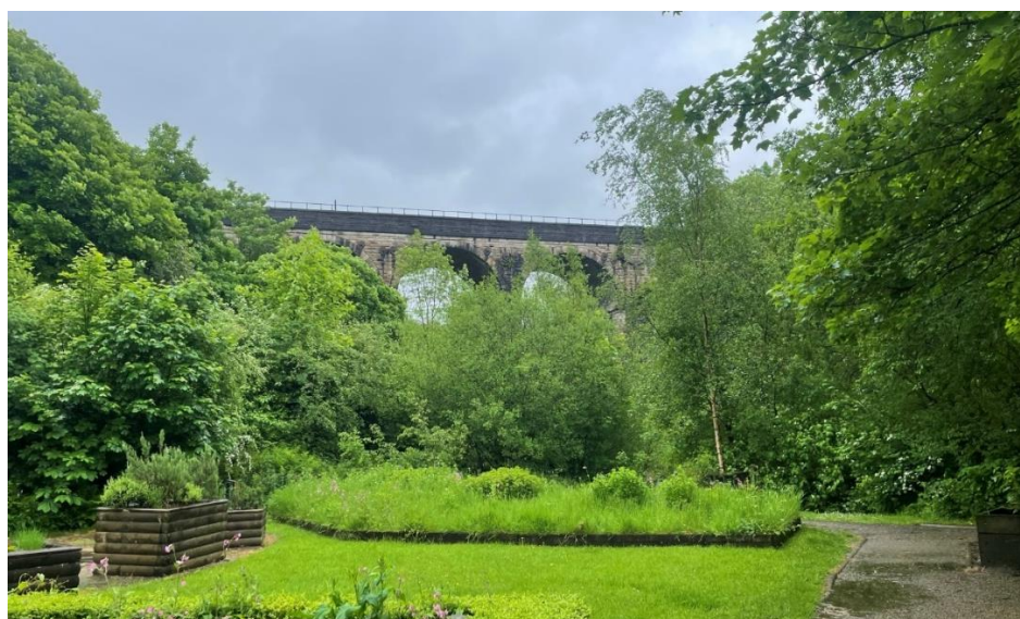
Insert 5-9 View of Uppermill Viaduct (MVL3/31) from the Brownhill Nature Garden to the north, showing an example of a restricted view of the structure.
