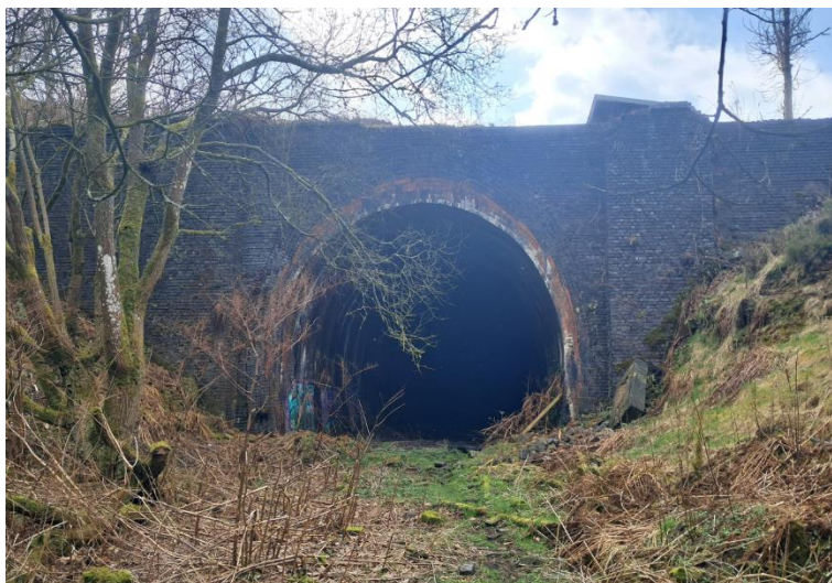
The north entrance to Butterhouse Tunnel. March 2025.
