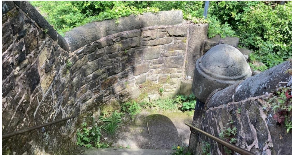
Insert 5-6 Springbank Lane Footbridge (MVL3/8), curved approach from the east.
