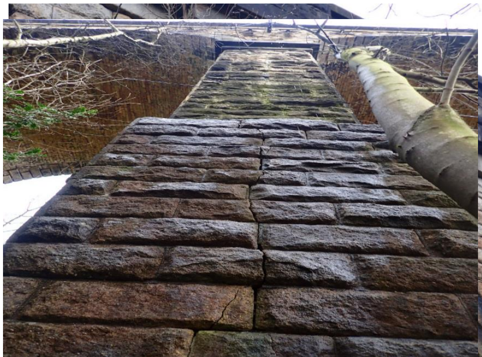
Insert 1-3 Example of typical vegetation around one of the downpipe hoppers.
