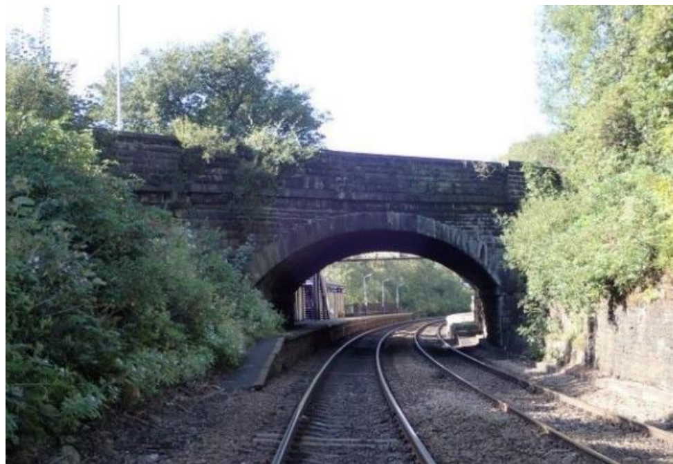
Insert 5-4 Oldham Road Overbridge (MVL3/28) north-east elevation
