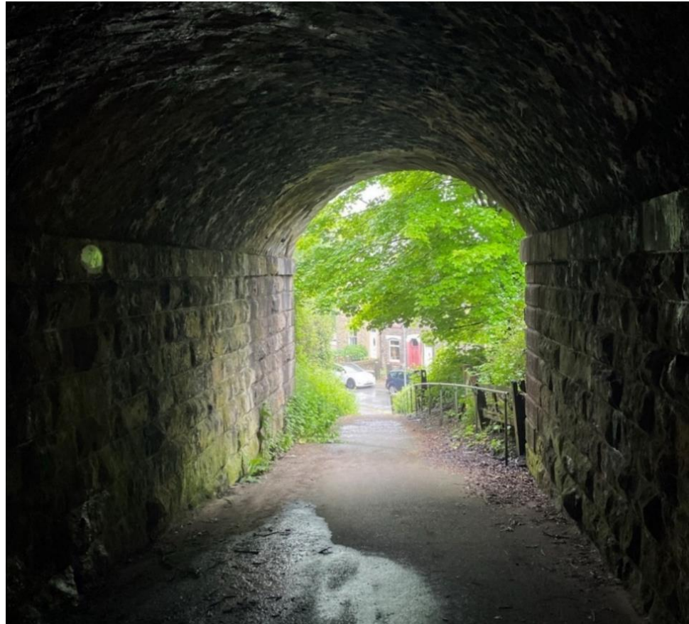
Insert 5-4 Shaw Hall Bank Road Footway (MVL3/26) looking south towards Shaw Hall Bank Road.
