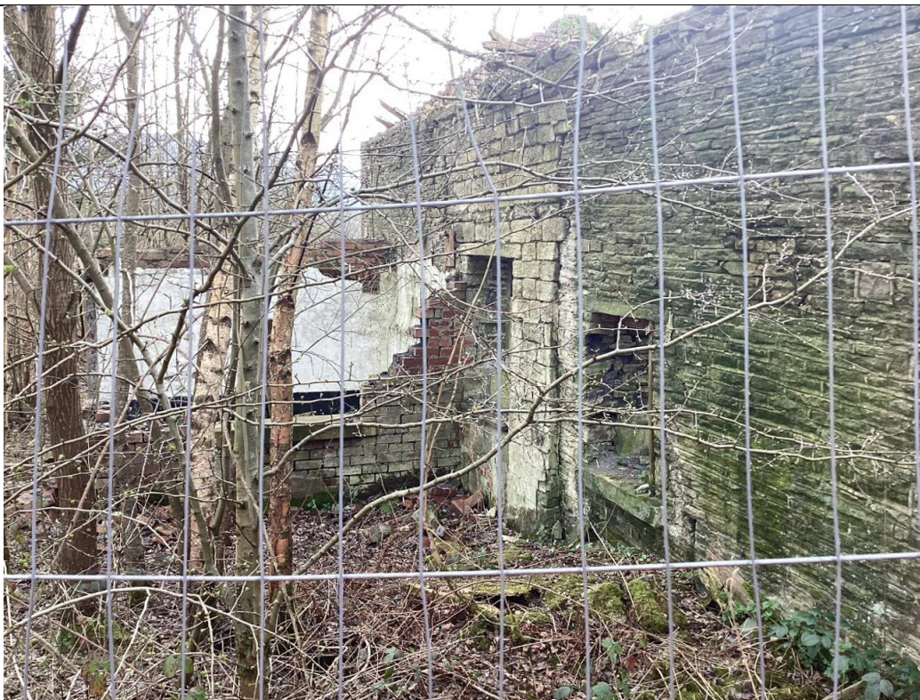
Principal (north) elevation of the barn at Printworks Office Compound
