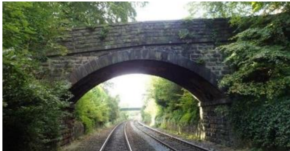
Insert 5-3 Heyrod Hall Overbridge (MVL3/7) north-east elevation.
