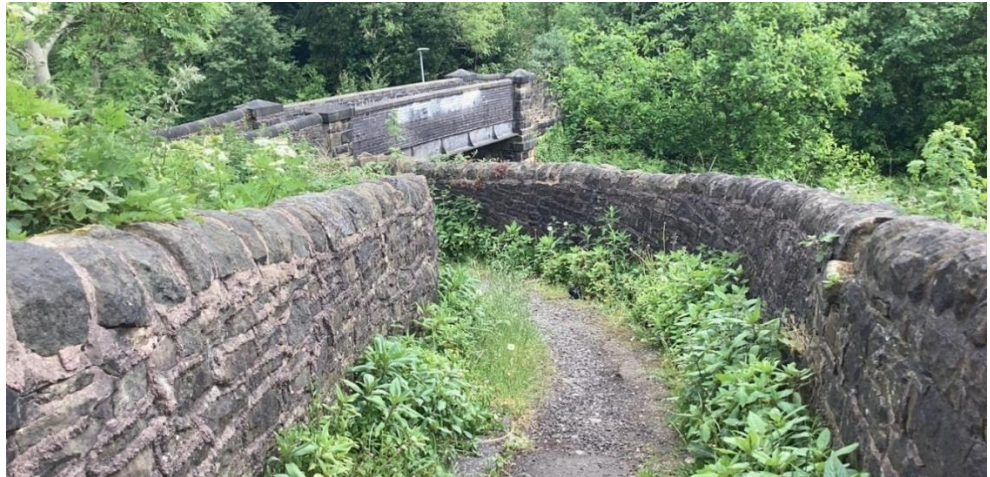
Insert 5-7 Springbank Lane Footbridge (MVL3/8), approach from Wakefield Road to the west of the overbridge.
