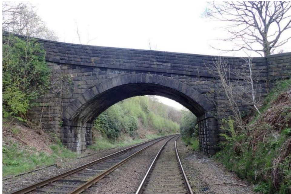
Insert 5-2 Wright's Overbridge (MVL3/23), south-west elevation.
