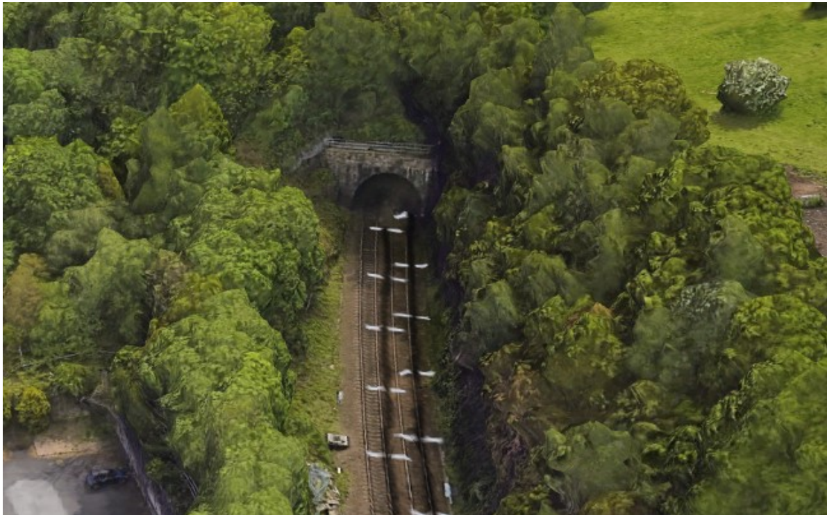
Figure 1-4 - Scout Tunnel – Northern Portal. Off A635 Manchester Road.
