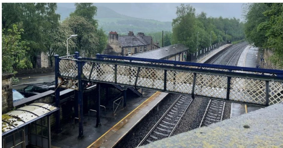
Insert 5-7 Oldham Road Bridge (MVL3/28), looking south-west overlooking the railway alignment. Greenfield Station Footbridge (MVL3/27A) is visible
