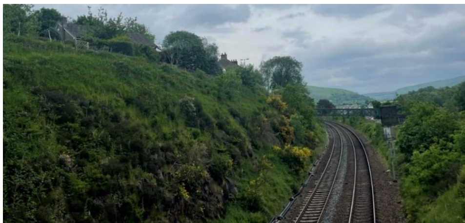
Insert 5-12 Roughtown Road Overbridge (MVL3/17), view looking north-east from the across the bridge deck.
