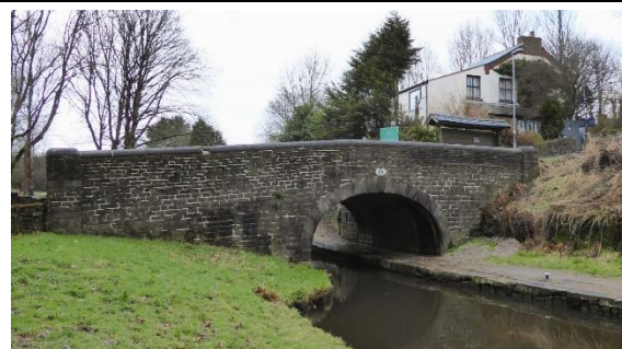
Huddersfield Narrow Canal No. 66 Bridge
