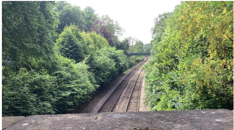
Insert 5-5 Heyrod Hall Overbridge (MVL3/7), view across the bridge parapet looking north-east
