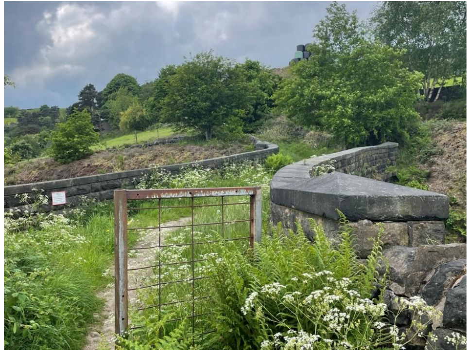
Insert 5-10 View east across the deck of Wright's Mill Overbridge (MVL3/20).
