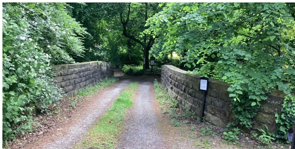
Insert 5-4 Heyrod Hall Overbridge (MVL3/7), view south-east across the bridge towards Heyrod Hall.
