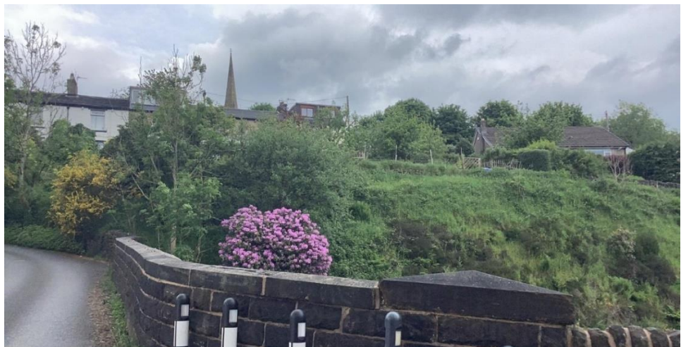
Insert 5-15 Roughtown Road Overbridge (MVL3/17), looking west from the end of the bridge deck with the spire of St John the Baptist Church visible.
