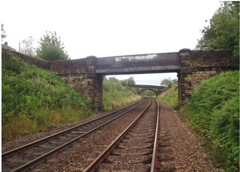
Insert 1-1 Springbank Lane Footbridge (MVL3/8) south elevation in the foreground
