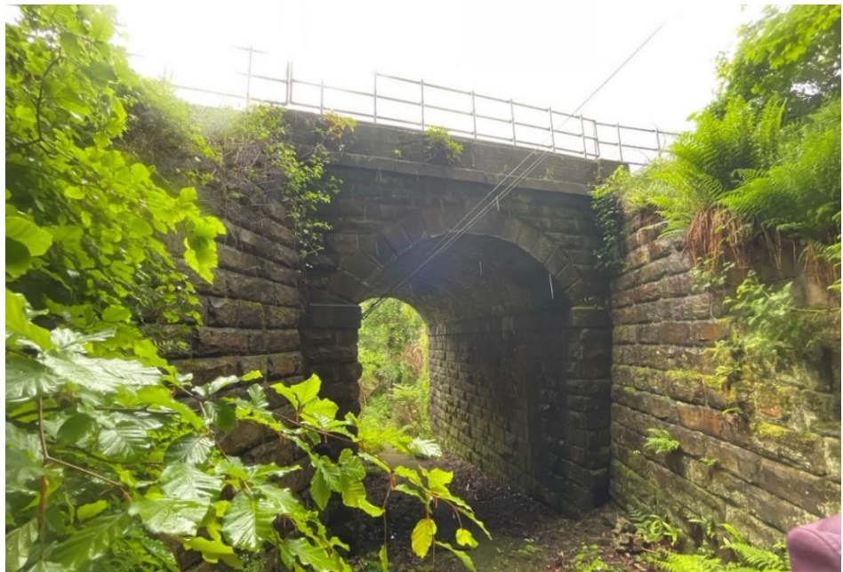
Insert 5-4 Wickens Underbridge (MVL3/29) west elevation.
