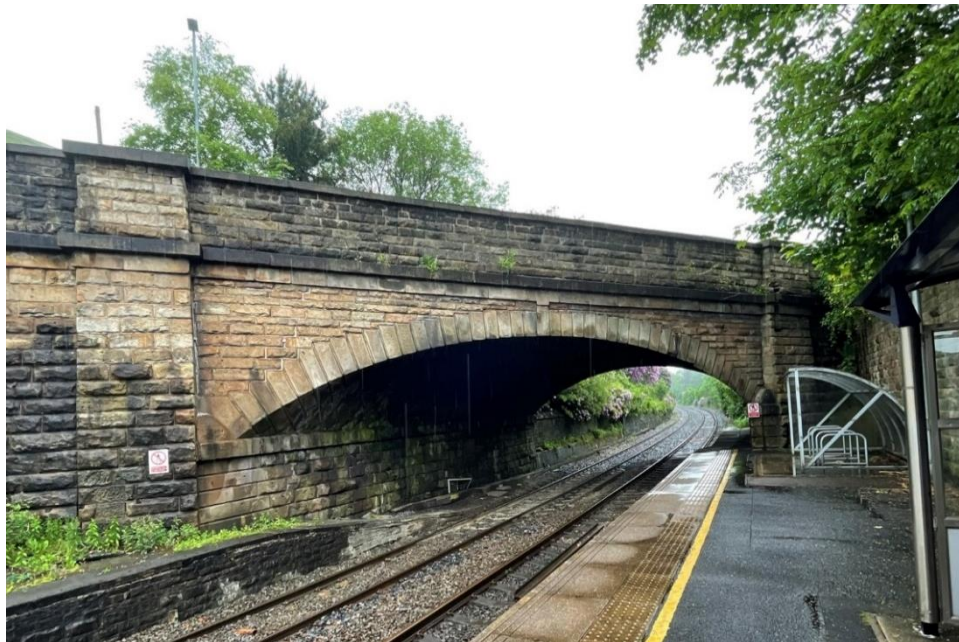
Insert 5-5 Oldham Road Overbridge (MVL3/28) south-west elevation from Greenfield Station.
