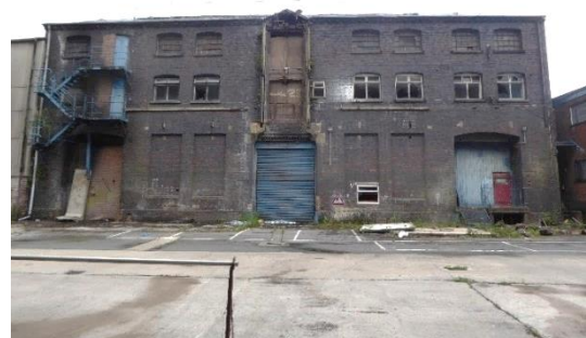
Micklehurst Loop goods warehouse at Plevins
