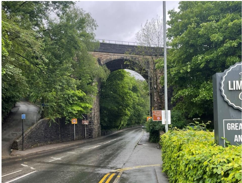
Insert 5-10 View of Uppermill Viaduct (MVL3/31) from Wool Road.
