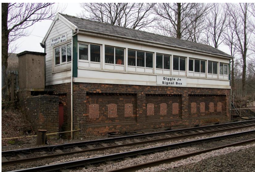
Diggle Junction Signal Box (LNW, 1885), located outside the compound boundary.
