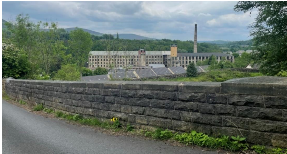
Insert 5-14 Roughtown Road Overbridge (MVL3/17), looking east from the end of the bridge deck with the former Cotton Mill (now Warmco Woodend Mill) in the distance.
