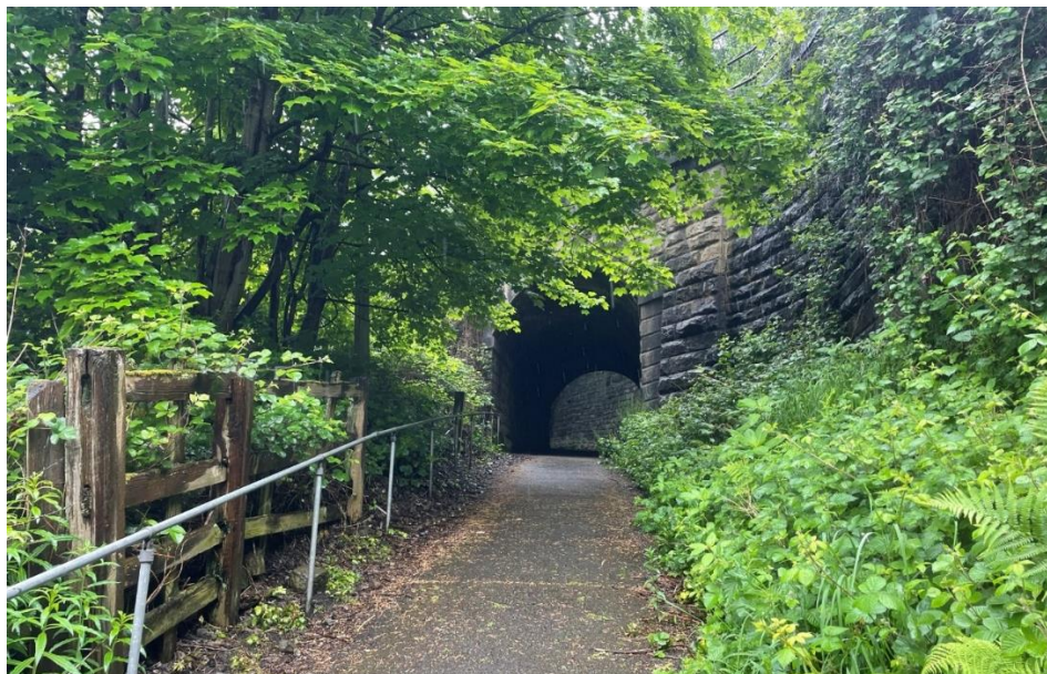
Insert 1-1 Shaw Hall Bank Road Footway (MVL3/26) south elevation.
