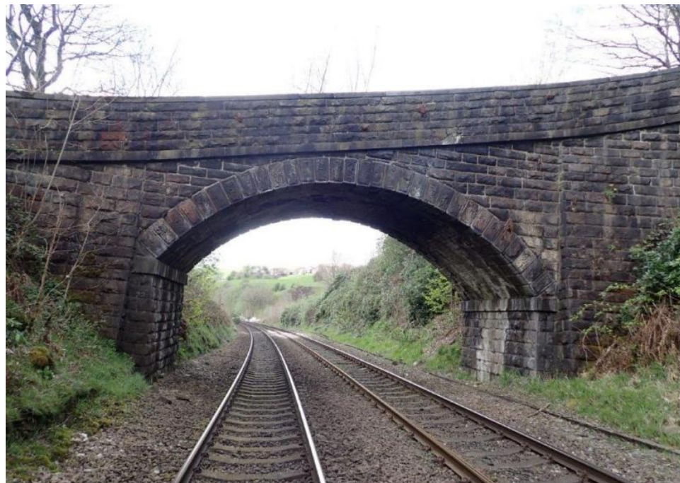
Insert 5-3 Wright's Overbridge (MVL3/23), north-east elevation.
