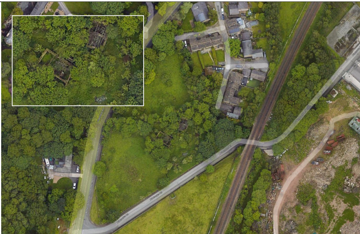
Aerial image showing extant structures within proposed compound location. Base Map: Google Earth 2025
