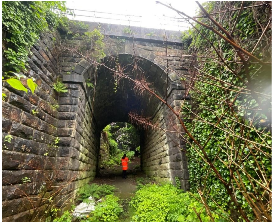
Insert 5-3 Wickens Underbridge (MVL3/29) east elevation.
