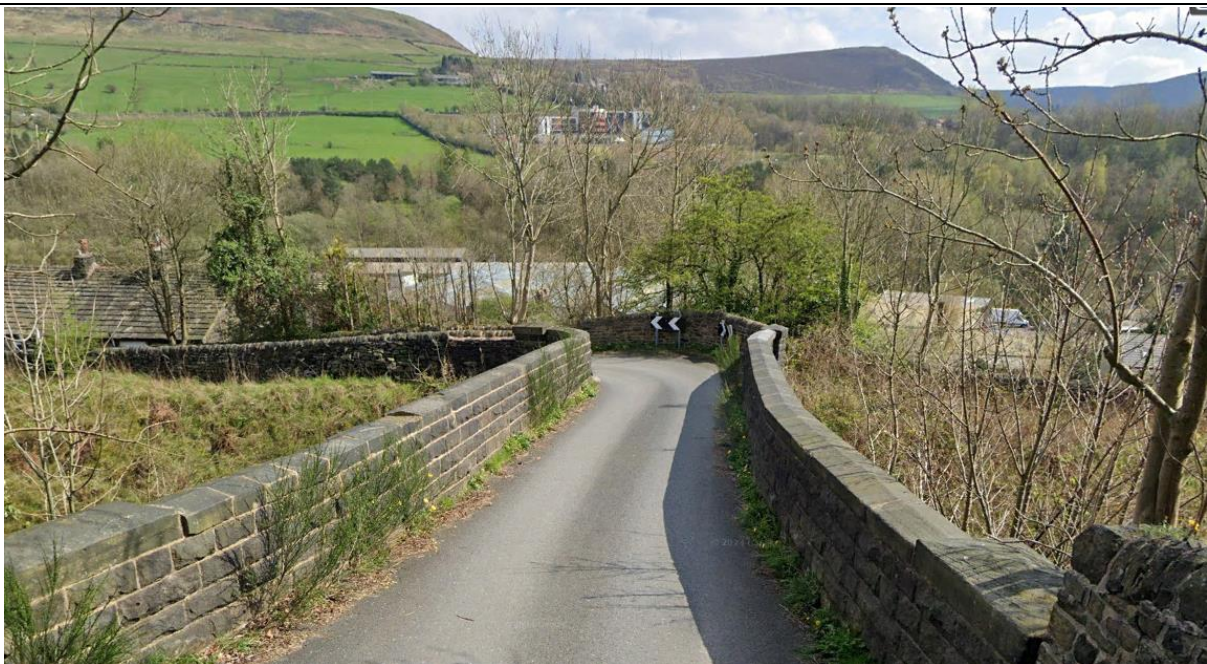
GoogleStreetView of Roughtown Road Overbridge, looking west
