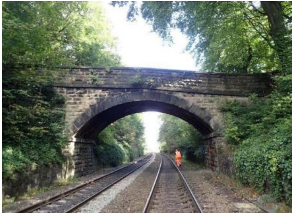
Insert 1-1 Low mileage (south-west) elevation of Heyrod Hall Overbridge (MVL3/7).
