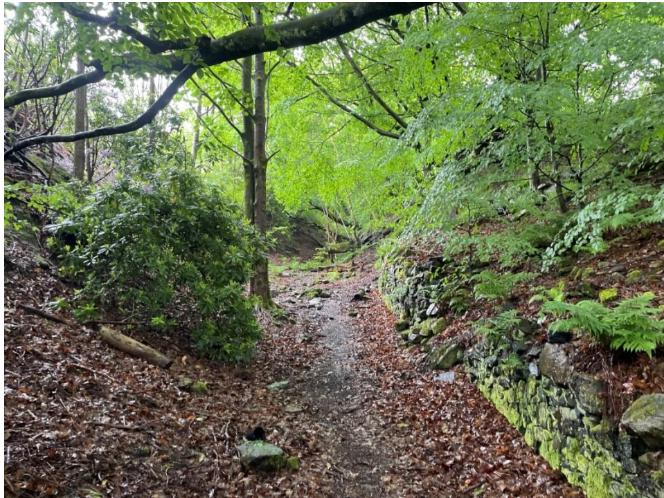
Insert 5-5 The setting of Wickens Underbridge (MVL3/29) looking west.
