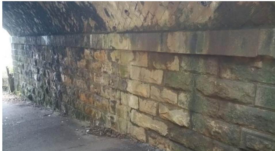
Insert 1-3 Shaw Hall Bank Road Footway (MVL3/26), soffit and masonry walling.
