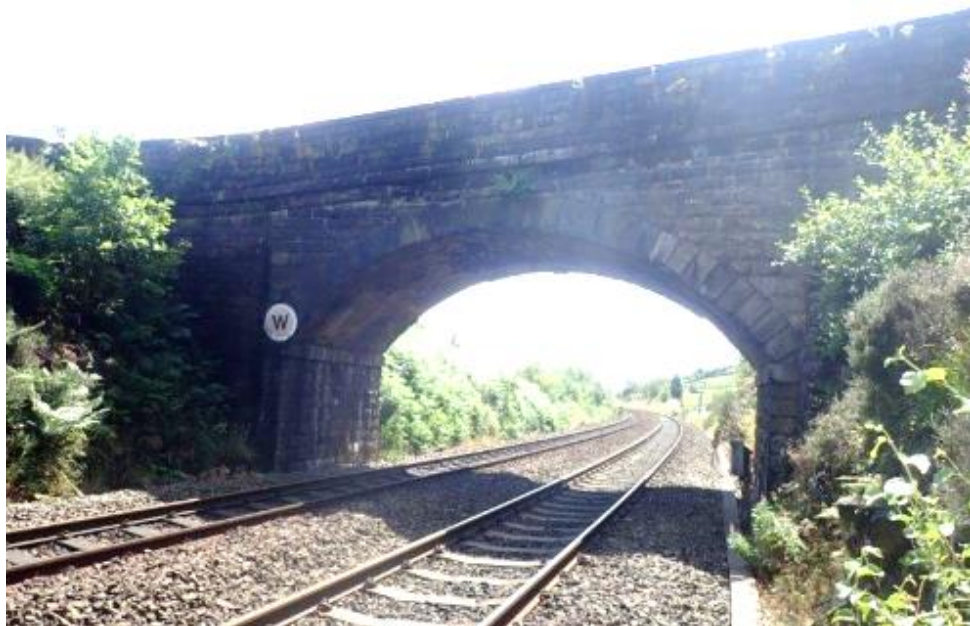
Insert 5-9 Wright's Mill Overbridge (MVL3/20), north elevation (Network Rail, 2022).
