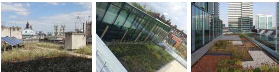
Figure 10.8 Green roofs (courtesy Sky Garden, Arup)
