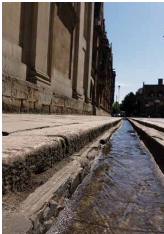
Figure 10.18 Roadside rills, Cambridge (courtesy Cambridgeshire County Council)
