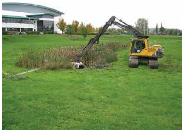
Figure 32.2 De-silting (courtesy Bedford Group of Drainage Boards)
