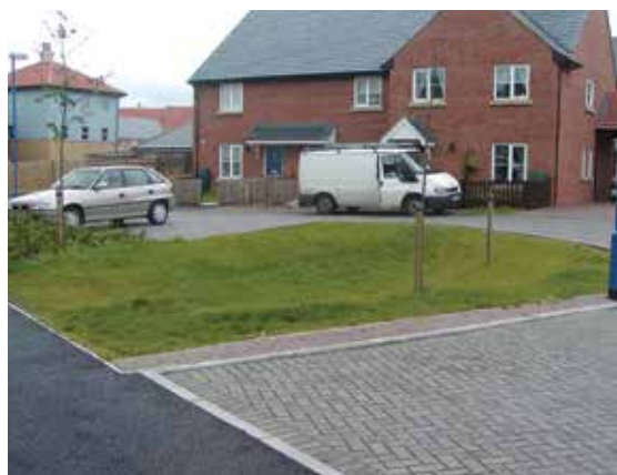
Figure 13.7 Small infiltration basin, Cambourne (courtesy Illman Young)
