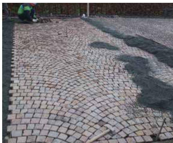
Figure 20.2 Private driveway using natural stone as permeable paving (courtesy The Ethical Stone Company/SteinTec)
