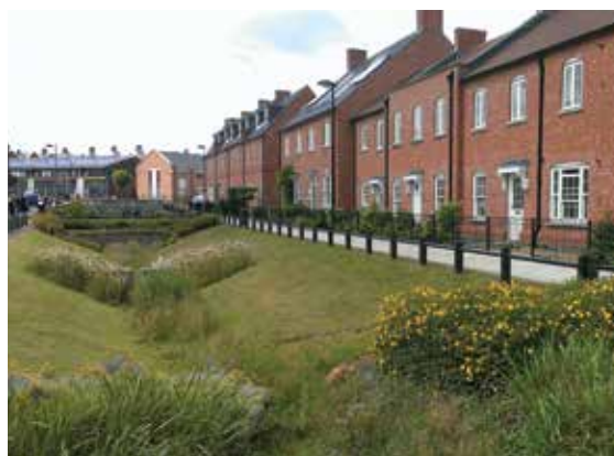
Upton, Northamptonshire (courtesy Peterborough City Council)
