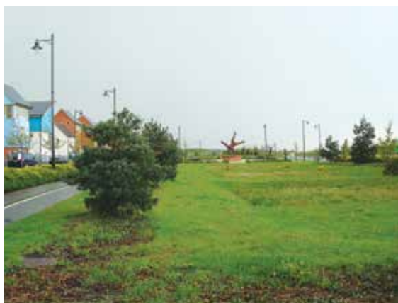
Figure 13.6 Large infiltration basins, Ipswich (courtesy Graham Fairhurst)
