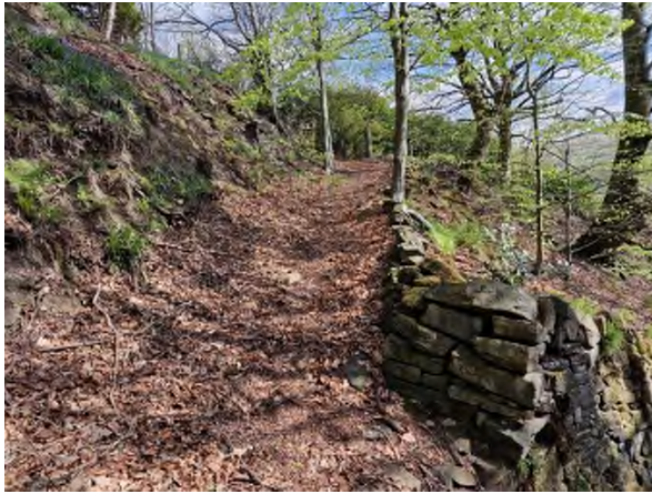
Photo 5.8e – Section of Public Footpath (looking West, uphill)
