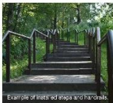
Example of metal ad steps and handrails.
