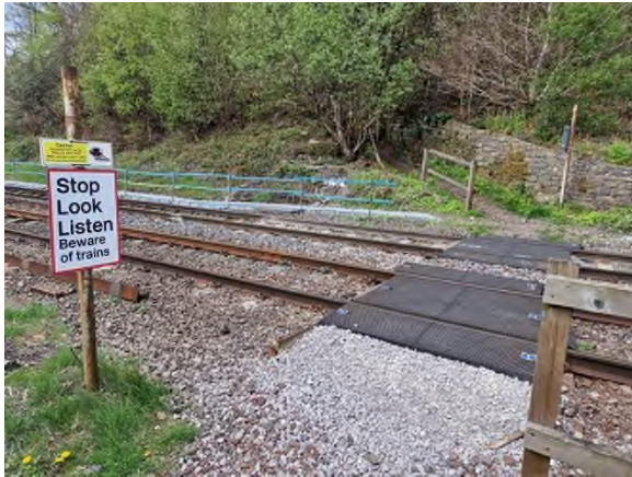
Photo 2.7b – Level Crossing (looking West)
