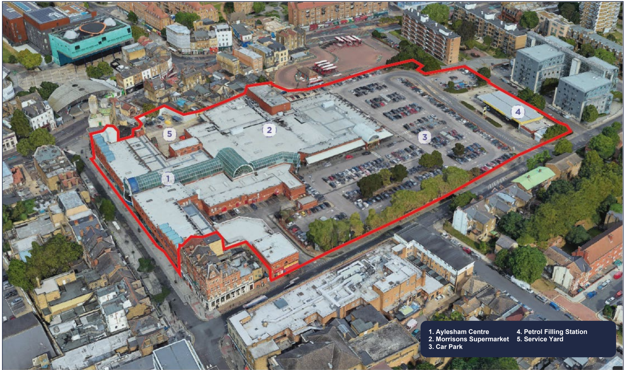
Aerial View of Current Site Condition
