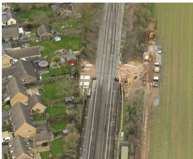
Figure 3 – Temporary footbridge being constructed and built
