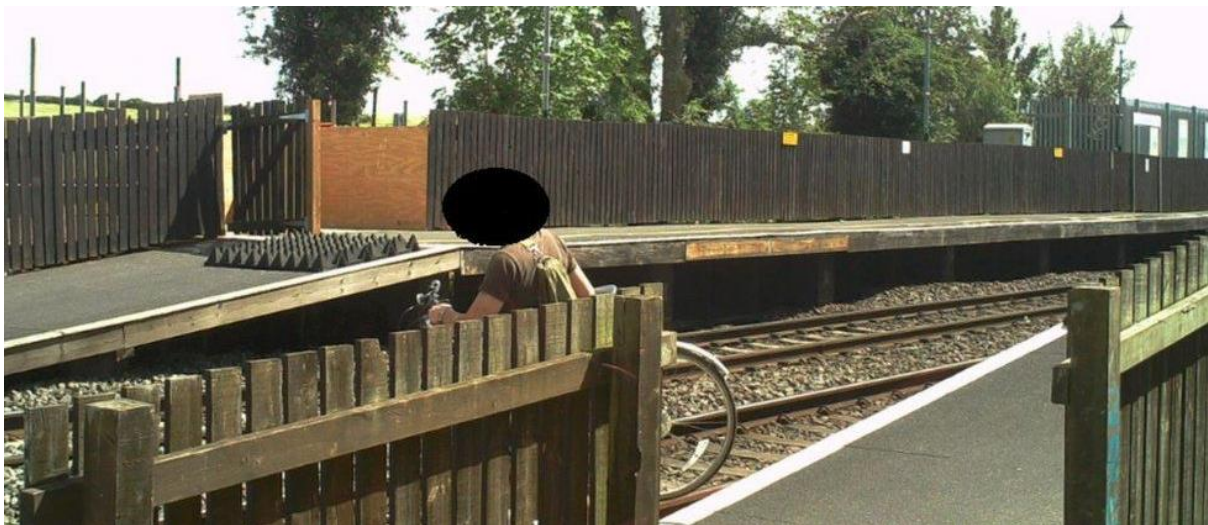
Figure 15: A cyclist seen walking over the tracks between platforms, despite the temporary footbridge being in place. (BBC, 2020).
