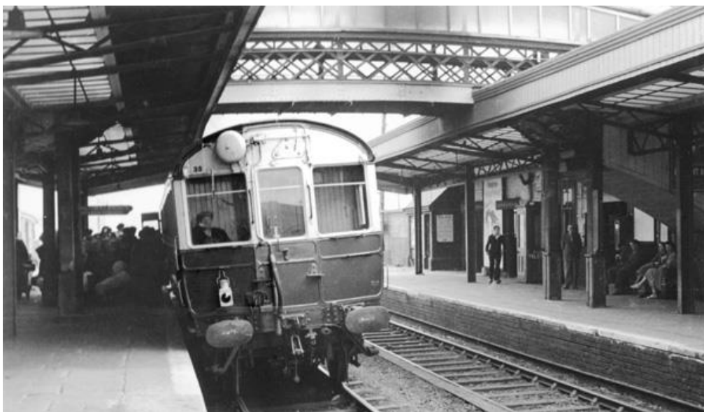
Figure 12: Photo of Banbury station taken in 1952, prior to its modernisation. The original lattice footbridge can be seen overhead. (The Patrick Kingston Collection, as viewed on the Steve Banks website, 1952).
