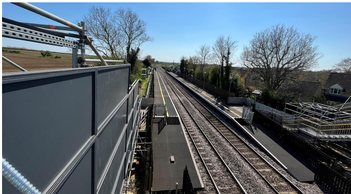
Figure 10: View from the temporary footbridge looking south, showing the existing station arrangement.
