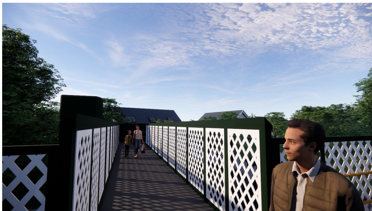
Figure 14: Partially transparent lattice parapets aid visibility for users.
