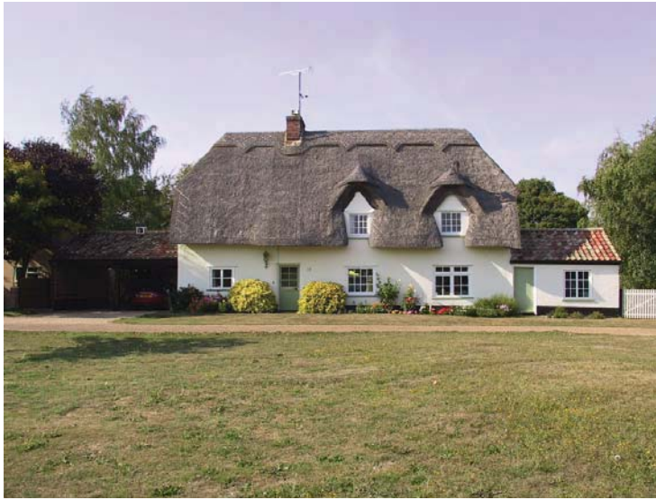
Extended cottage, Barrington. The openings of the right-hand extension balance the front cottage elevation, with painted render and a clay pantiled roof. The dark stained open timber frame of the left-hand carport helps it to recede from view.
