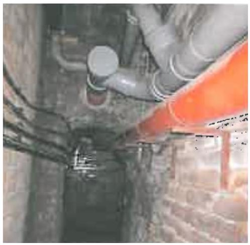
Figure 5.4.8.1c: Foul and roof water drainage within station cellar walkway
