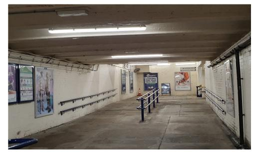
Figure 5.7.1.6a: Existing lighting scheme within the subway
