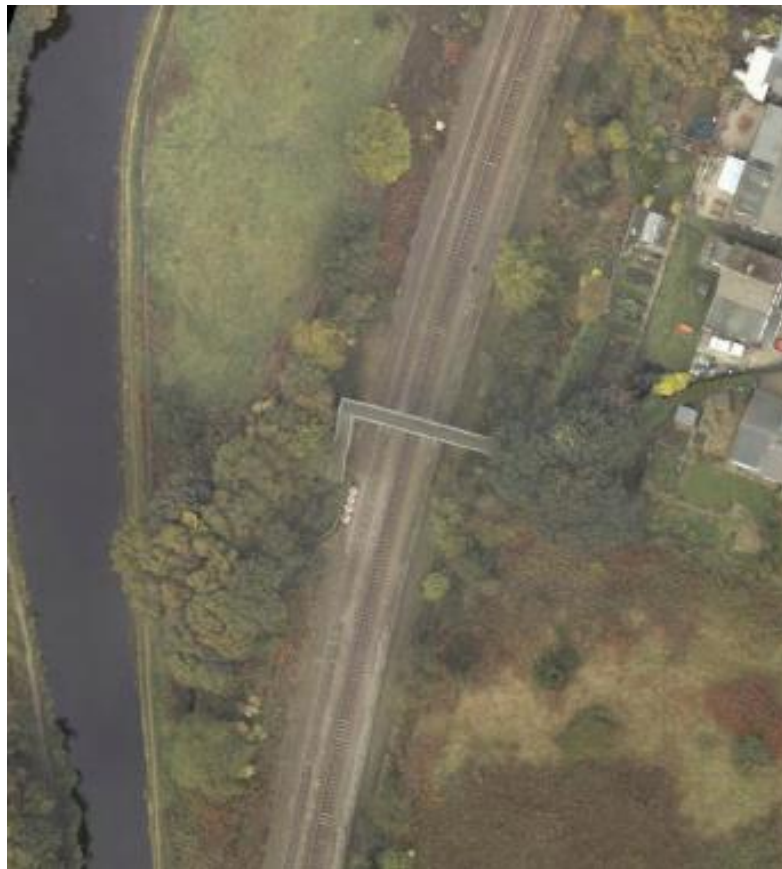
Figure 58: Ravenstone Drive Footbridge (MVL3/35) Aerial View
