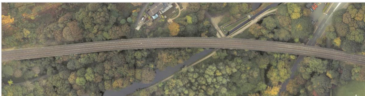
Figure 38: Uppermill Viaduct (MVL3/31) Aerial View
