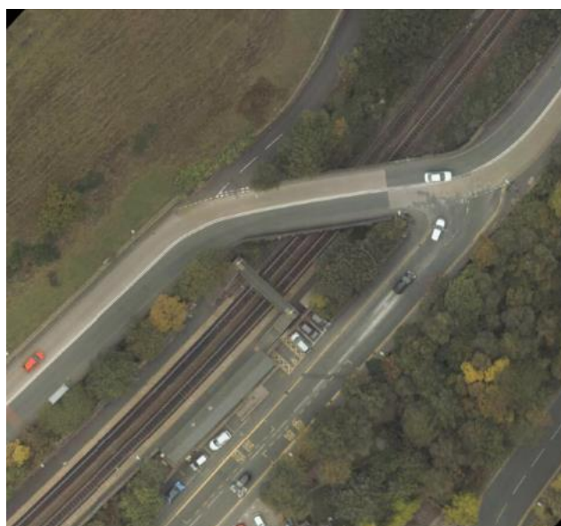
Figure 30: Oldham Road Overbridge (MVL3/28) Aerial View
