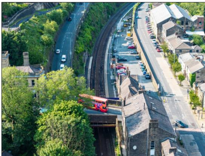
Figure 79: Mossley Station (Existing) Aerial View (facing north)
