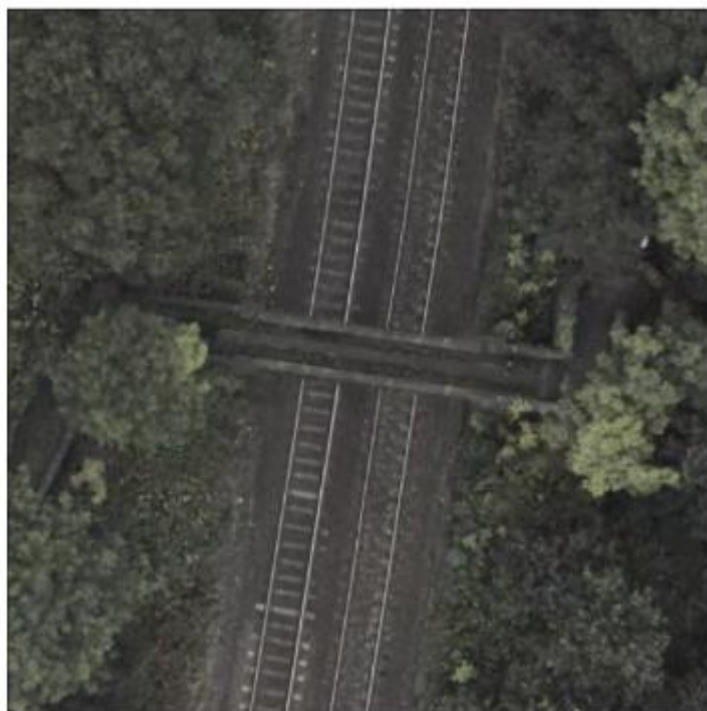
Figure 6: Springbank Lane Footbridge (MVL3/8) Aerial View
