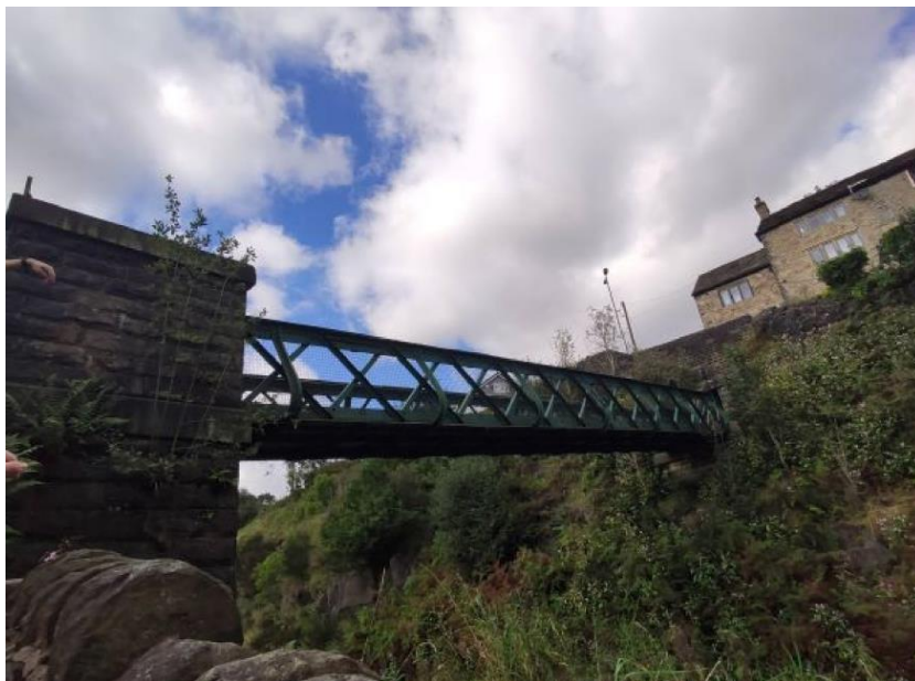
Figure 51: Rough Town Road Footbridge (MVL3/18) Existing High Mileage Elevation
