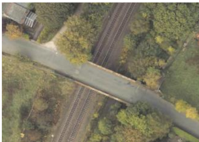
Figure 63: Ward Lane Overbridge (MVL3/26) Aerial View
