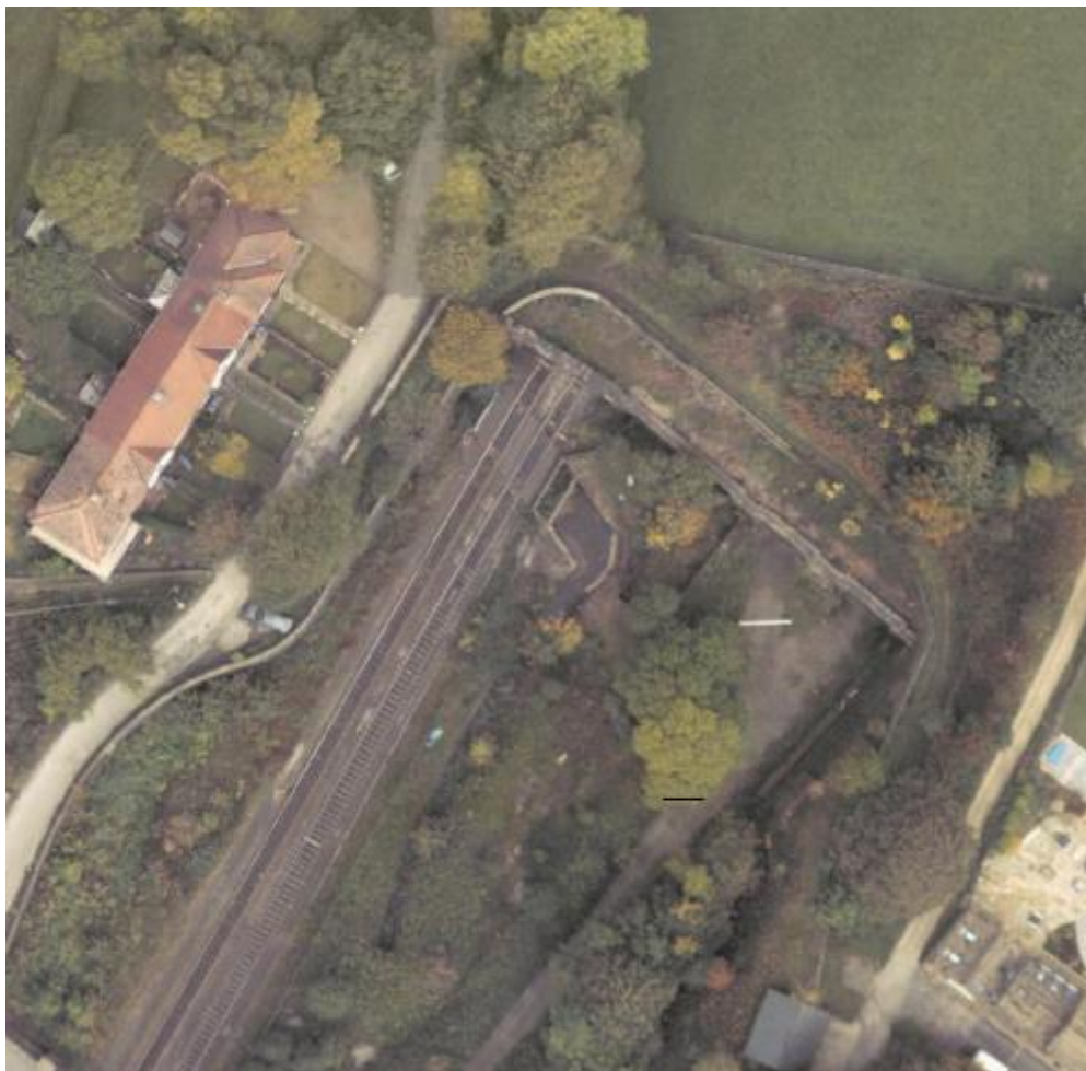
Figure 70: Bywash Underbridge (MVL3/39B) Aerial View
