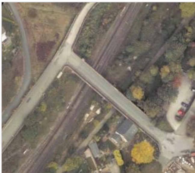
Figure 68: Station Road Overbridge (MVL3/39) Aerial View
