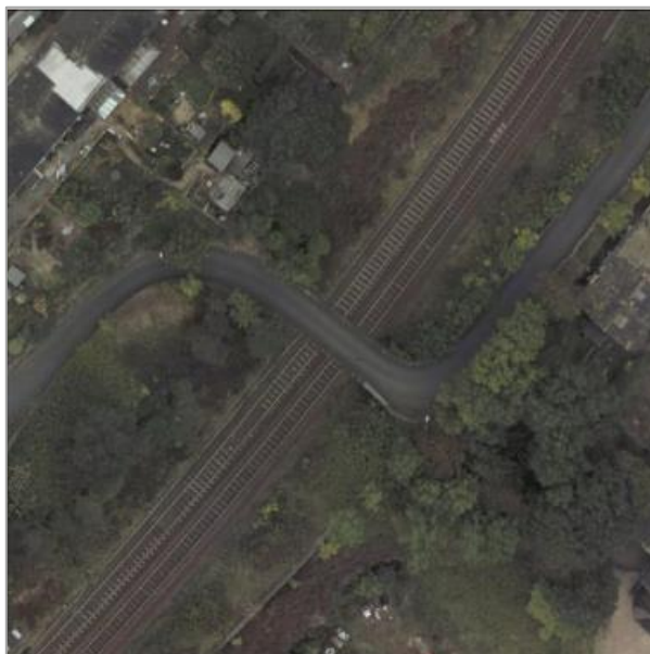
Figure 9: Roughtown Road Overbridge (MVL3/17) Aerial View
