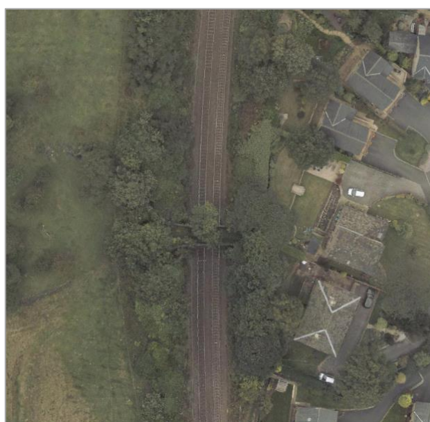
Figure 19: Wright's Overbridge (MVL3/23) Aerial View
