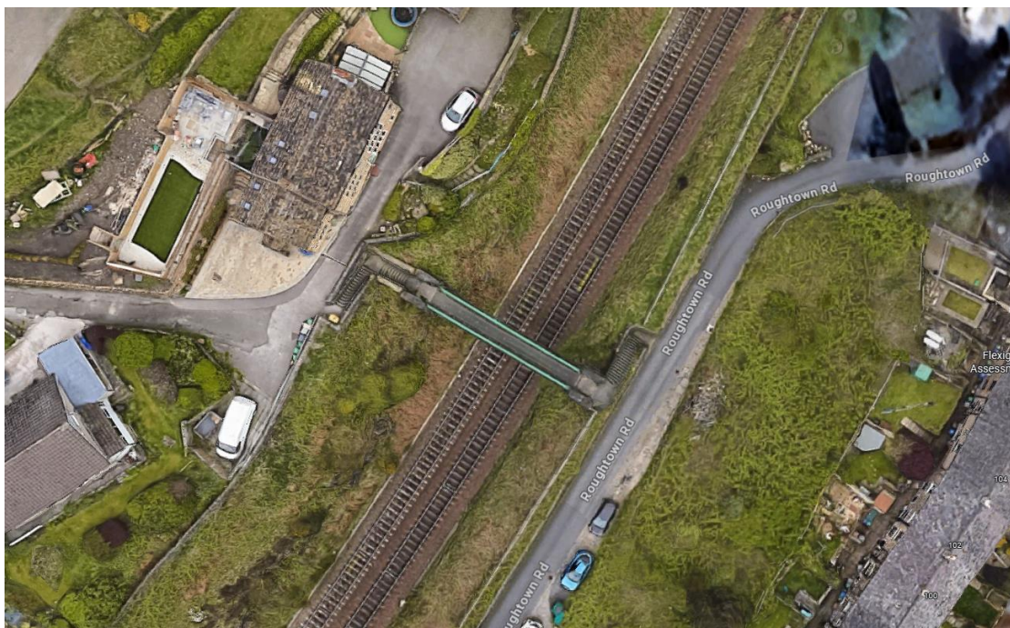
Figure 48: Rough Town Road Footbridge (MVL3/18) Aerial View
