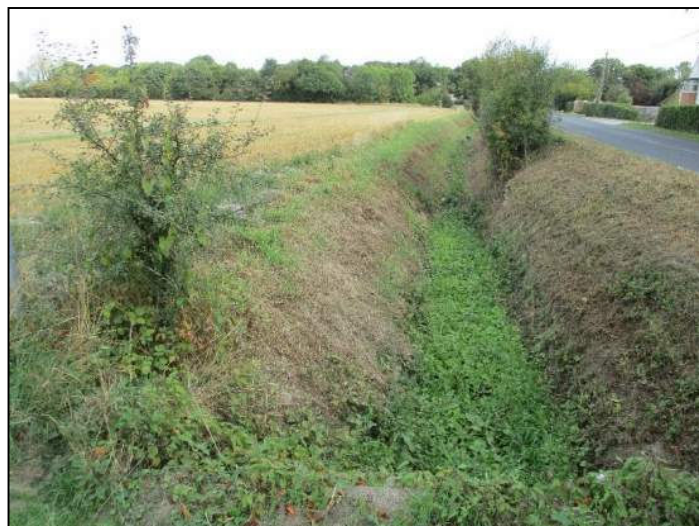
Photograph 12 - Ditch along Granham's Road (W22)
