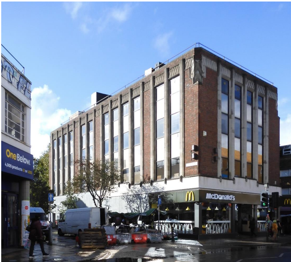
Precedent of vertical striped brick façade at 72 Rye Lane
