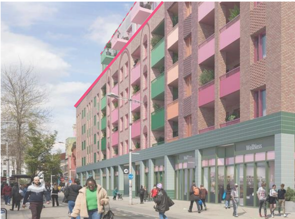
Building B is perceived as primarily five storeys along Rye Lane, with only partial visibility of the upper floors from street level.
