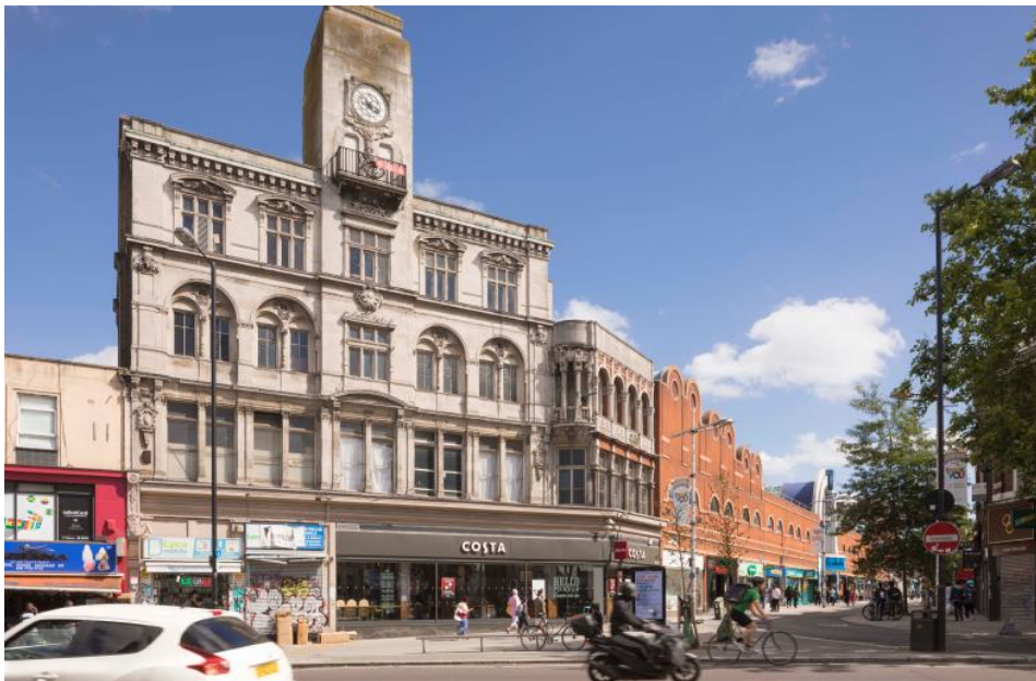
Key view from Peckham High Street (corner with Rye Lane) showing the existing building
