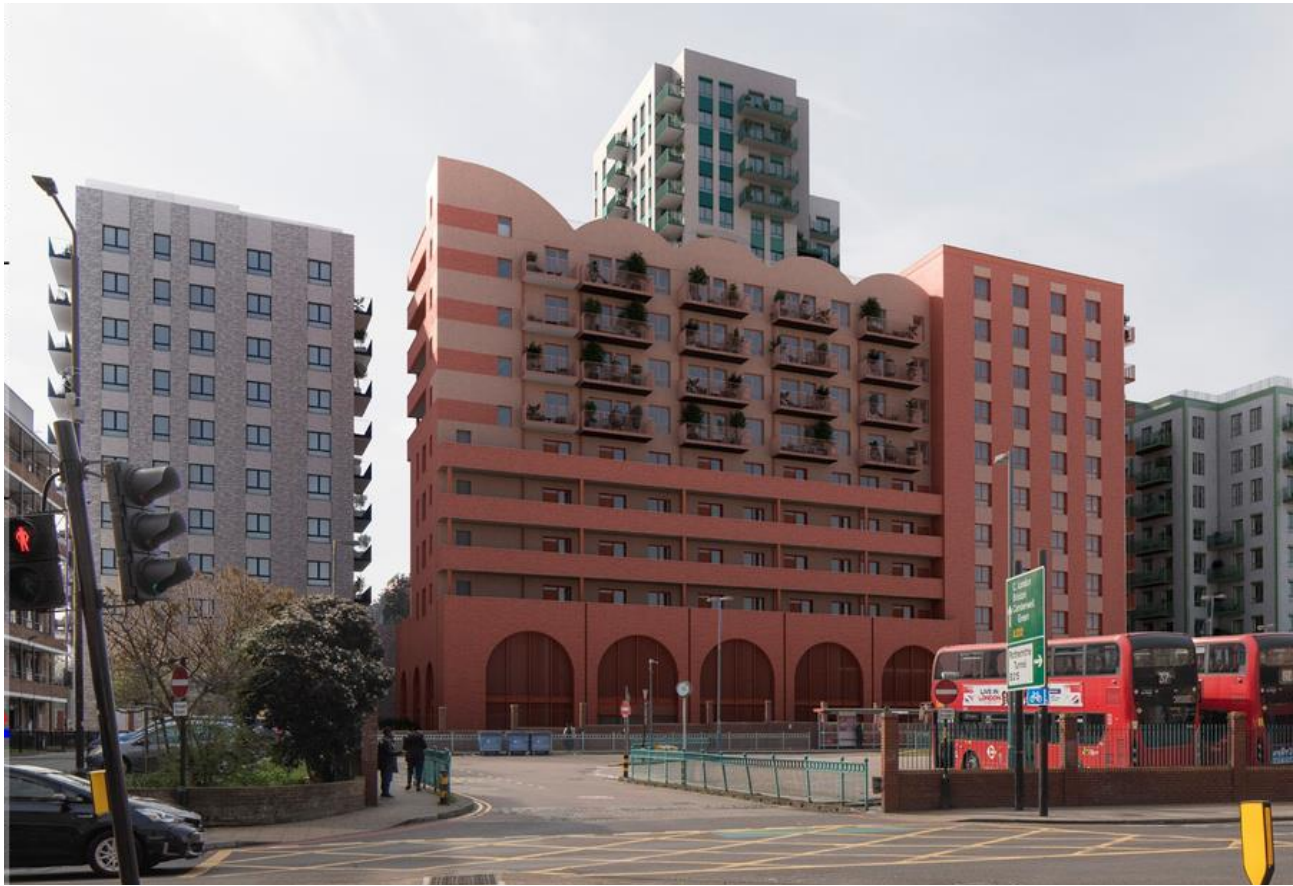
Building L North frontage to the Bus Station
