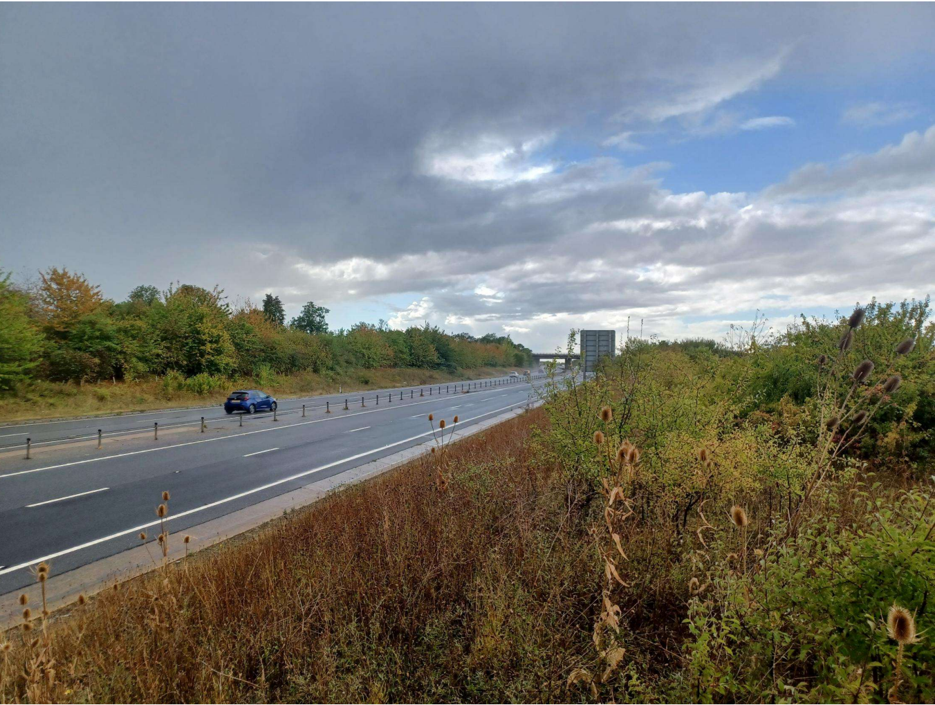
Plate 16: Photographs from Survey Location 4: Childerley A428 Camera Placements (looking west)
