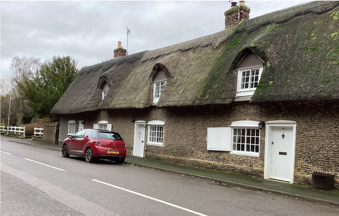
Figure A12.2.7 39 and 41 High Street
