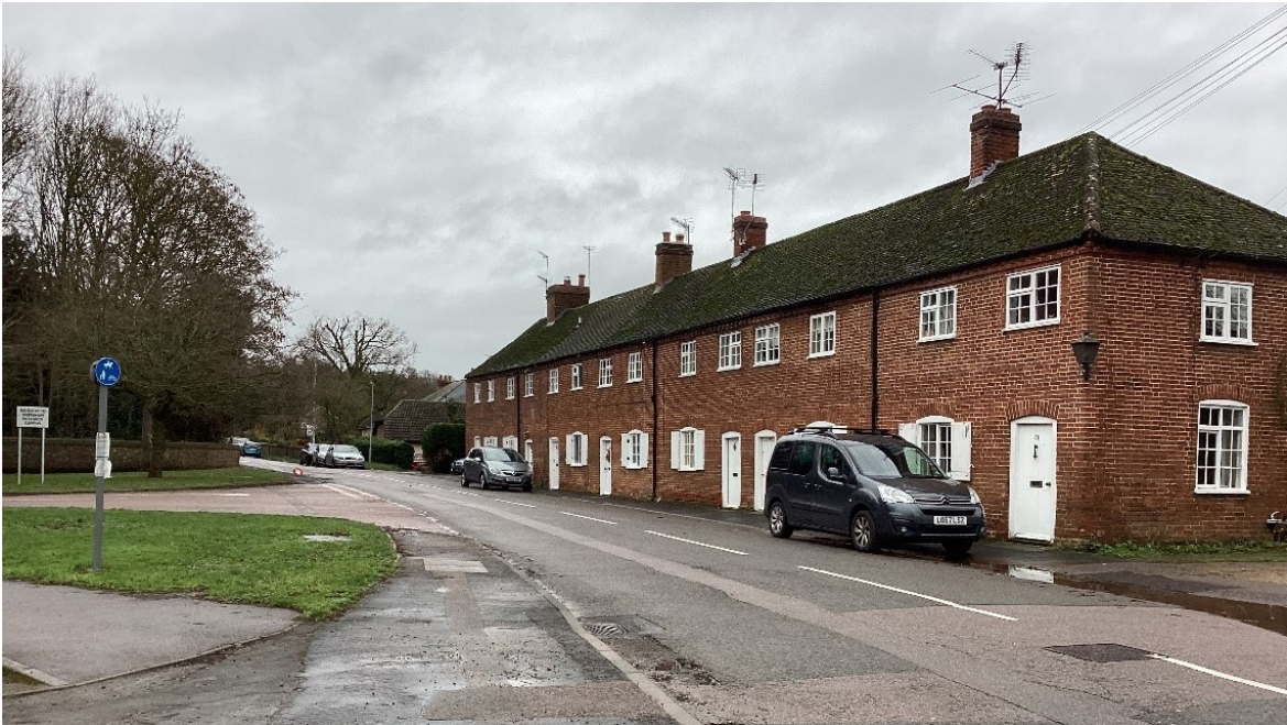
Figure A12.2.8 Brick Row
