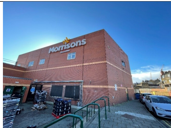
Photograph 12: Morrisons goods entrance boundary
