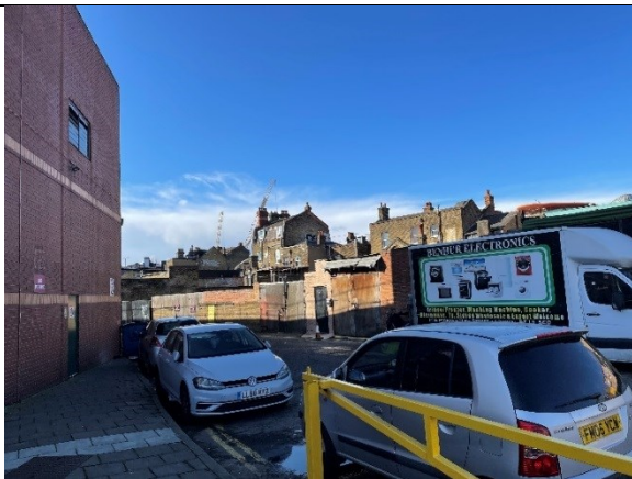
Photograph 11: Morrisons goods entrance
