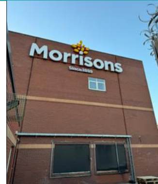
Image 10 External Brickwork - Morrisons
