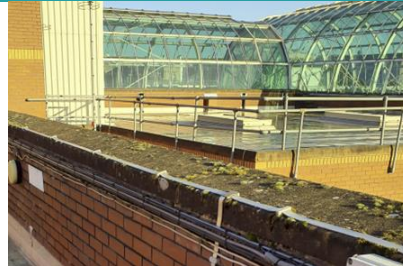
Image 12 Metal Handrails
