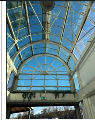
Image 30 Steel from Canopy
