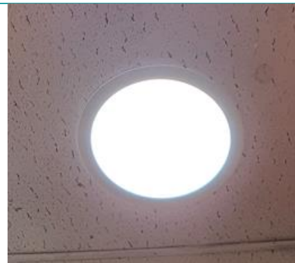
Image 111 Shopping Centre - Lighting
