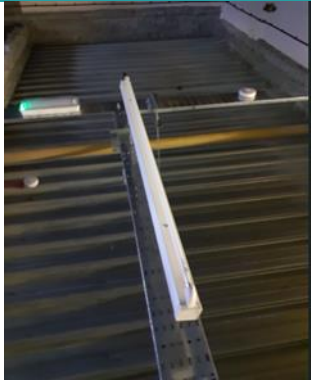
Image 19 Corrugated Metal Roof
