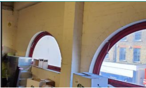
Image 15 Metal Window Frame
