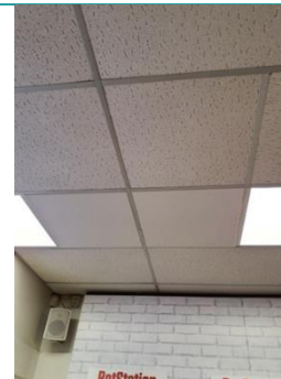
Image 63 Suspended Grid Mineral Tiles
