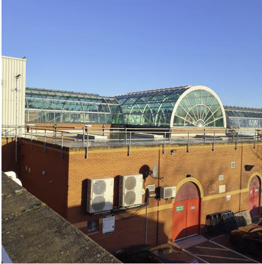
Image 1 Aylesham Centre – External from Roof
