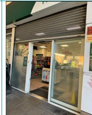
Image 18 Metal Window Frame and Roller Shutter
