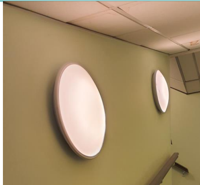
Image 118 Shopping Centre - Lighting
