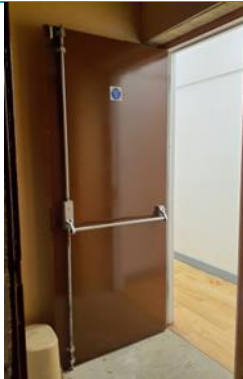
Image 41 Internal Timber Doors
