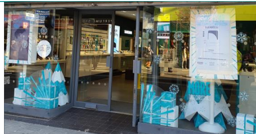
Image 16 Metal Window Frame
