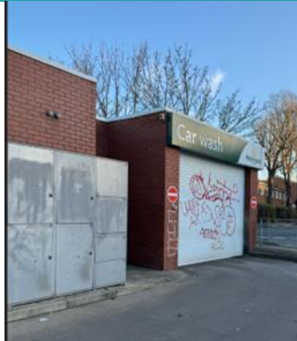
Image 9 External Brickwork - Car Wash
