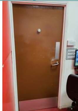
Image 42 Internal Timber Doors
