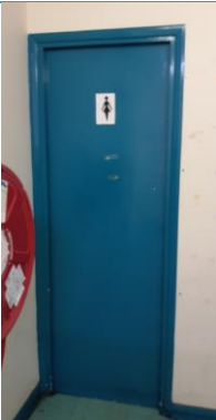
Image 40 Internal Timber Doors
