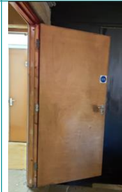
Image 43 Internal Timber Doors
