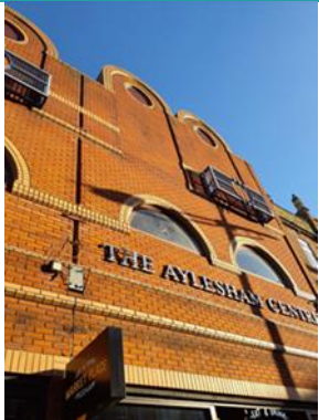
Image 8 External Brickwork - Aylesham Centre
