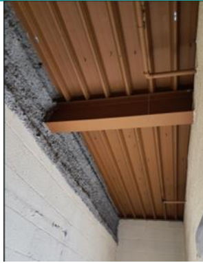
Image 20 Corrugated Metal Roof
