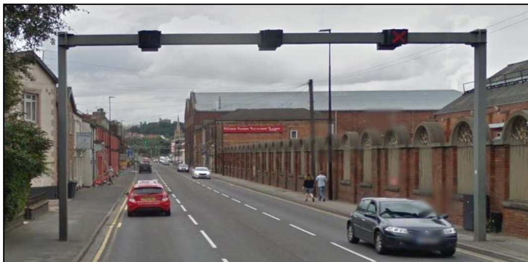
Figure 2: Northbound view of A15 Canwick Road
