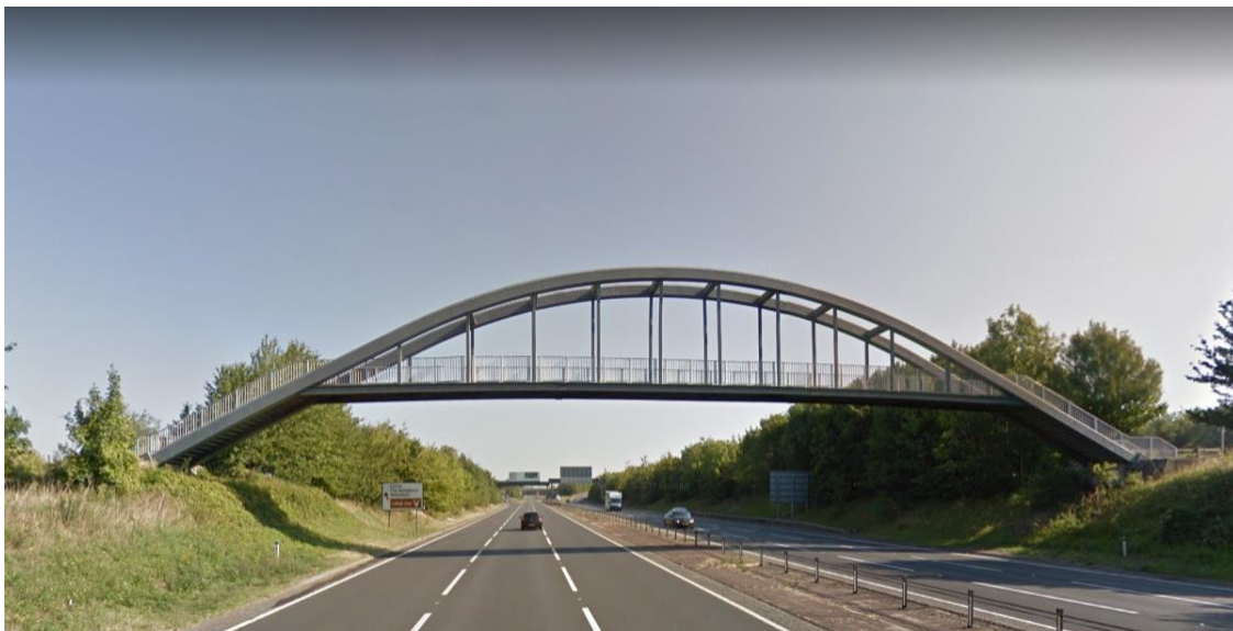
Figure 12.16: A11 Pedestrian Footbridge
