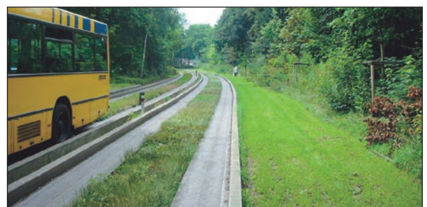
Figure 8.4 Guideway in Essen with central channel planting and landscaping
