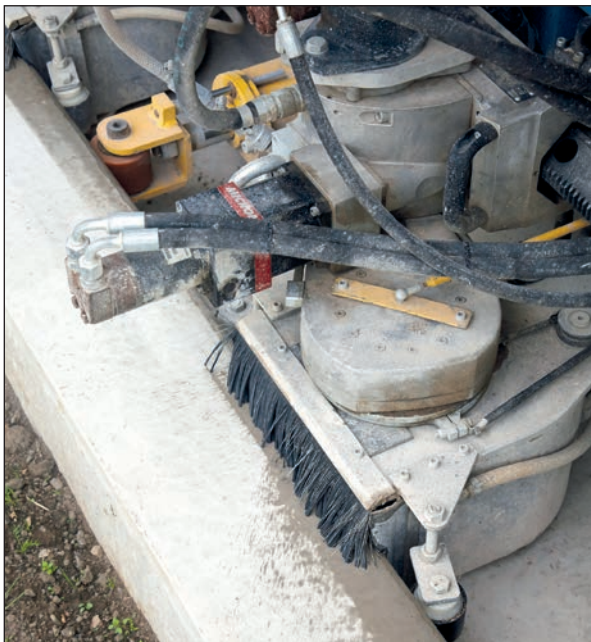
Figure 9.7 Grinding on Leigh & Ellenbrook busway
