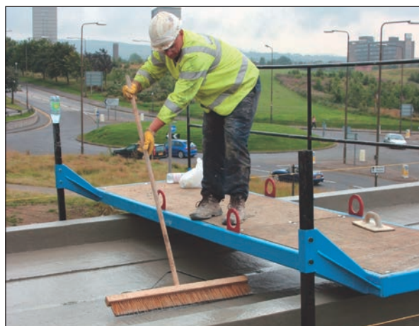
Figure 8.3: Transverse texturing on slip-formed guideway, Edinburgh
