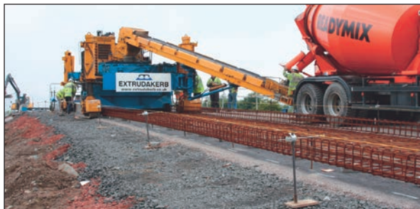
Figure 8.2: Reinforcement cage anchored into base slab, Edinburgh
