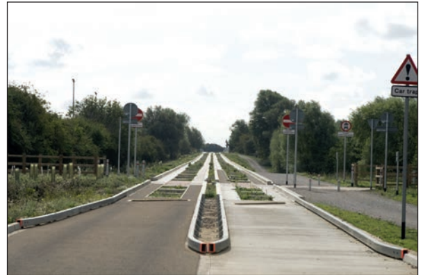
Figure 9.8 Cambridgeshire Guided Busway - steel guiderails for entry and exit splays
