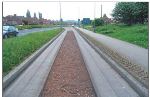
Figure 9.2 In situ concrete beams with precast kerbs, Leeds
