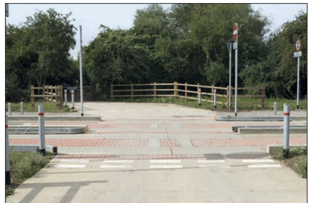
Figure 9.9 Burst through steel guiderails for entry and exit splays, Cambridgeshire
