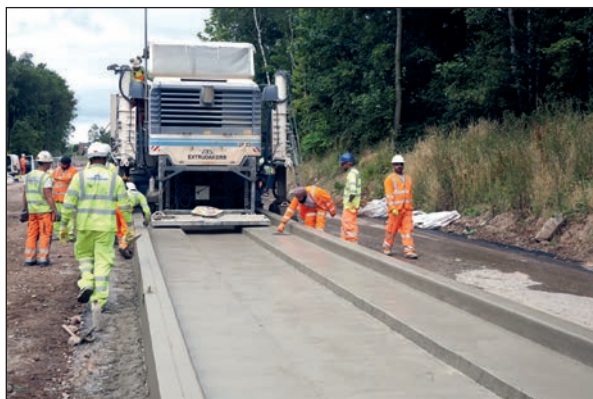
Figure 9.3 Slip-forming the Leigh to Ellenbrook Guided Busway
