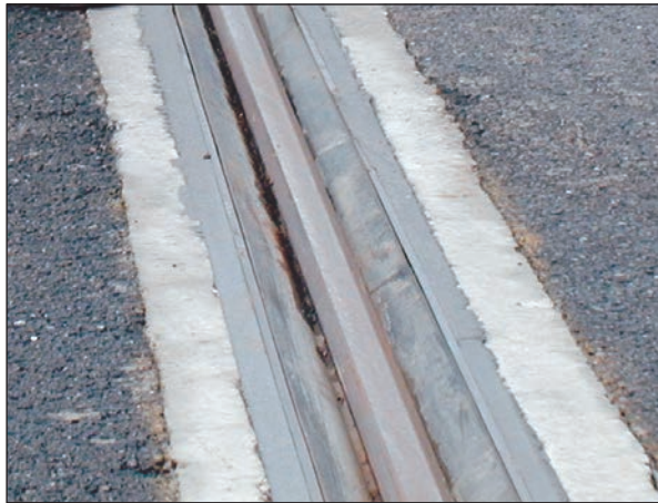
Figure 1.2 Translohr central guide slot
