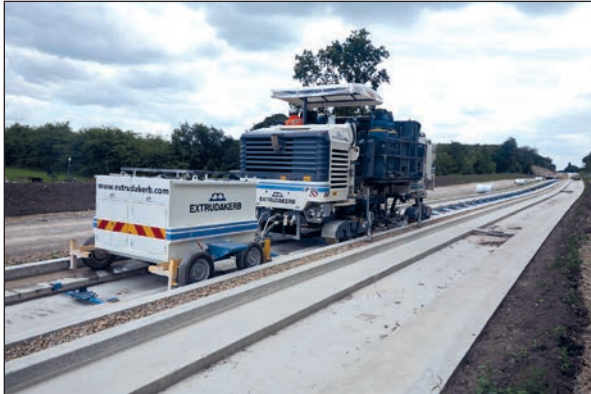
Figure 9.6 Leigh to Ellenbrook: Grinding the kerb
