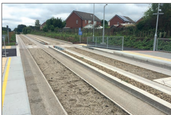
Figure 9.4 Leigh & Ellenbrook guideway with SuDS channels
