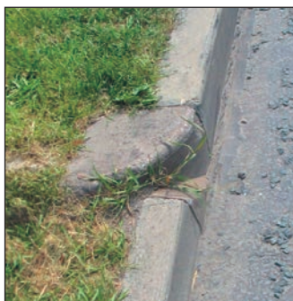
Figure 5.3 Quadrant kerbstone at step change in kerb height, Leeds
