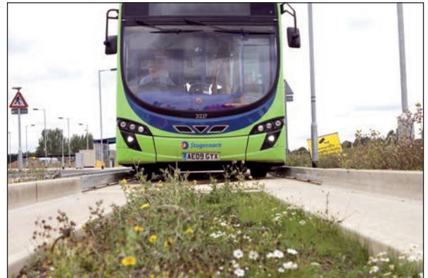
Figure 9.1 Buried precast concrete beams with infill, Cambridgeshire
