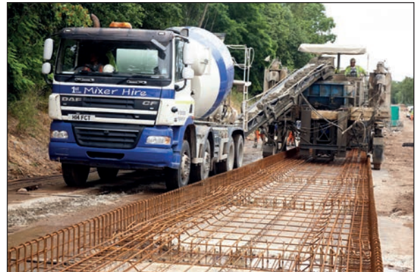
Figure 9.5 Leigh and Ellenbrook reinforcement cage
