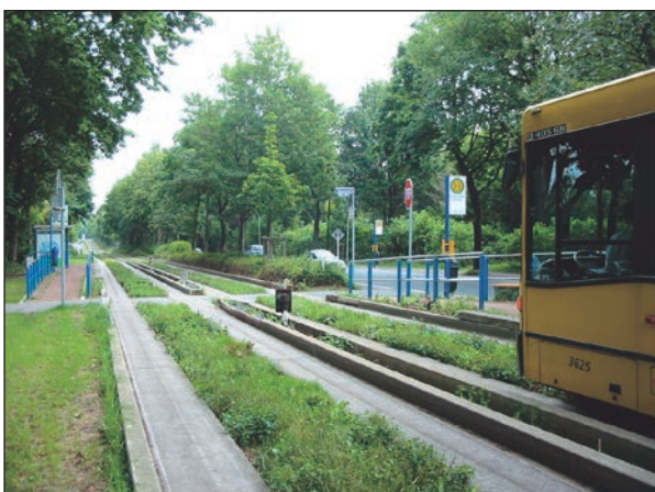
Figure 6.2 Staggered stop and pedestrian crossing, Essen
