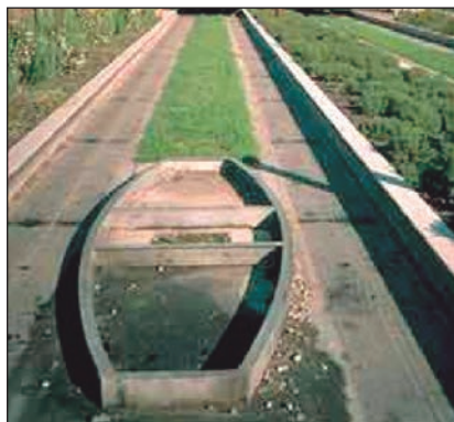
Figure 7.1 Example of a car trap at guideway entrance, Ipswich
