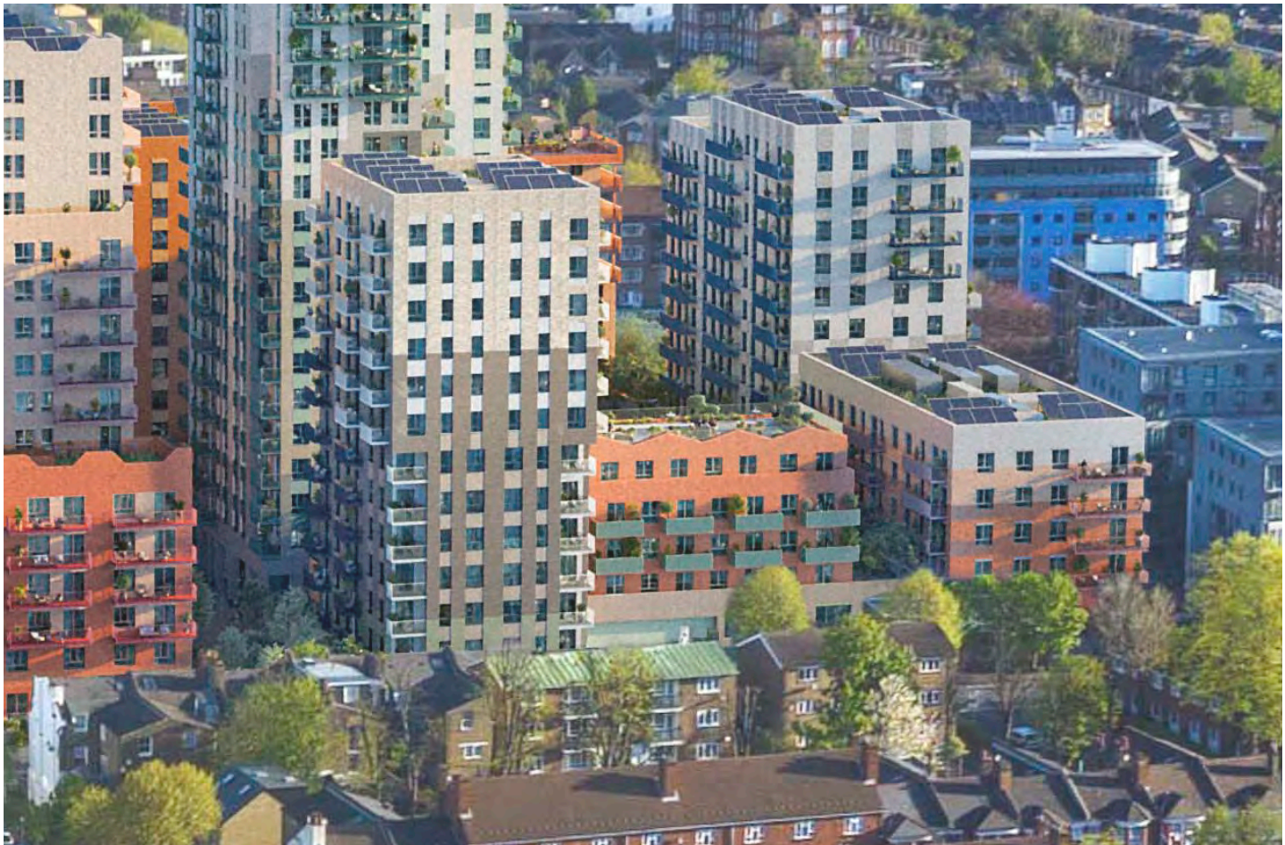
Aerial view of building N from south
