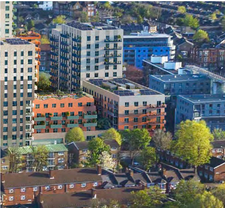
Aerial view of building Q looking north
