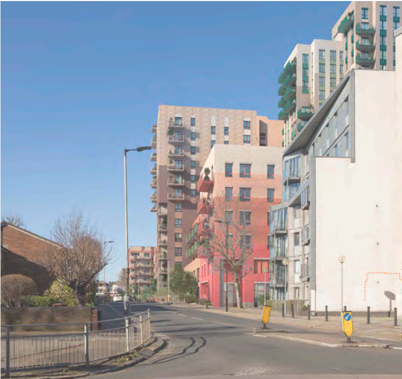
Building Q viewed from junction of Hanover Park and Clayton Road looking west
