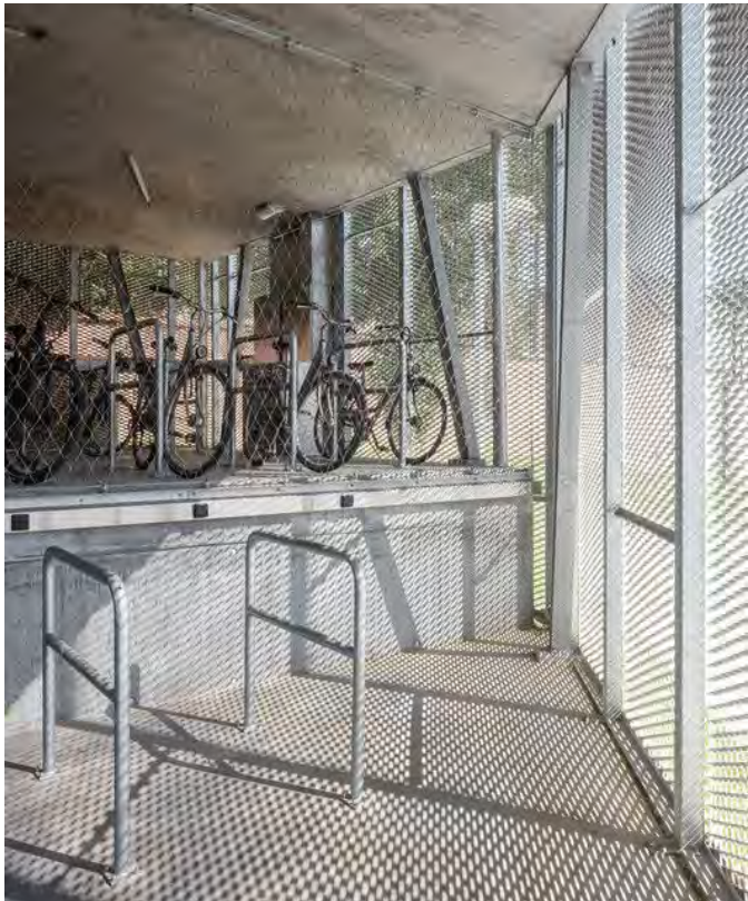
Cycle hub precedent - mesh allow natural lighting and ventilation
