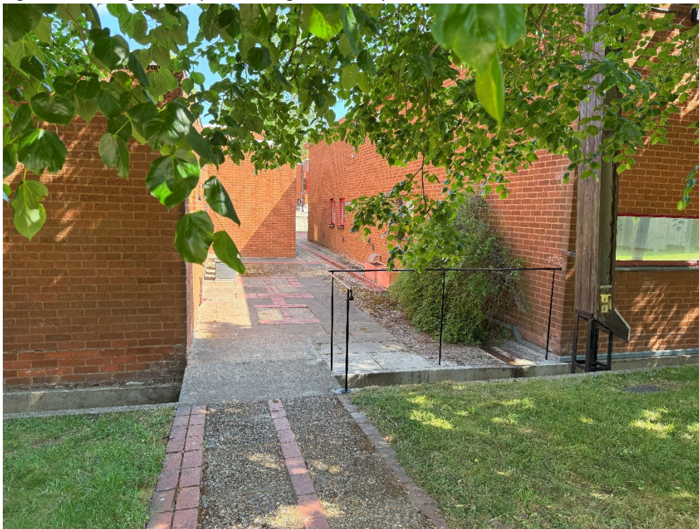
Figure 06 Existing view of path leading from Scholars' Walk
