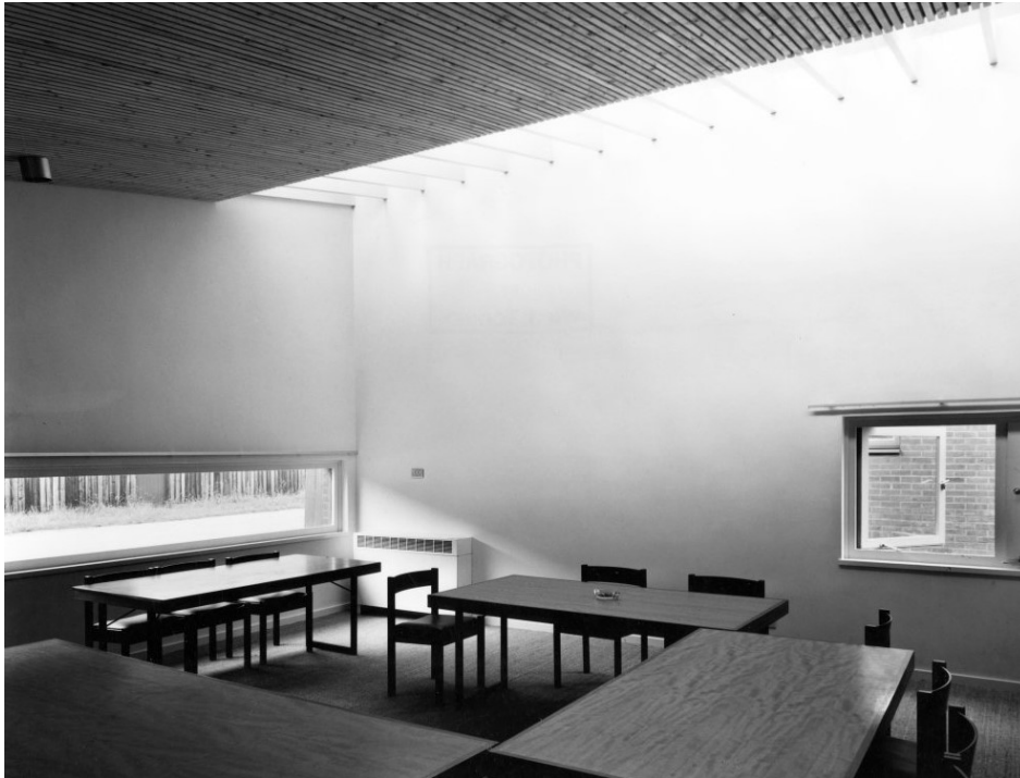
Figure 08 Original photo of meeting room showing relationship of window cill with seated position.
