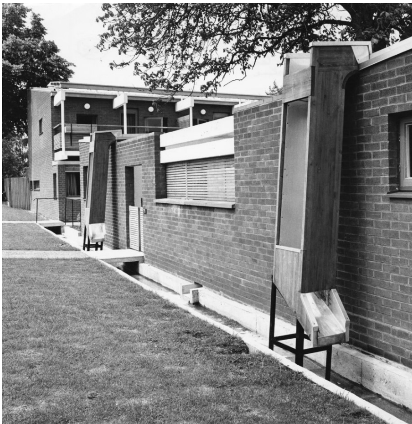
Figure 03 Original photograph looking towards the path leading from the courtyard house and Family Walk
