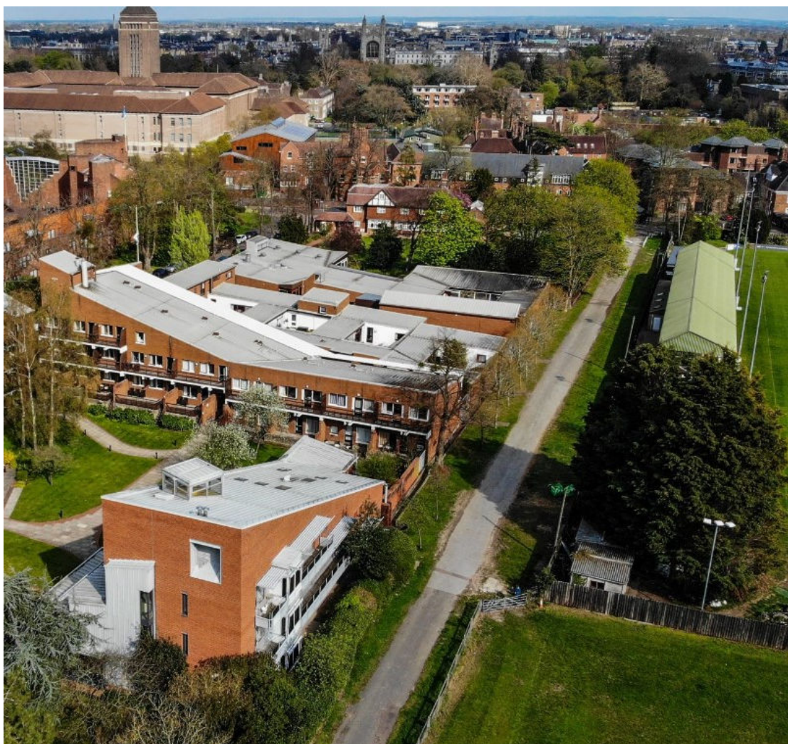
Figure 14 Aerial view of Clare Hall
