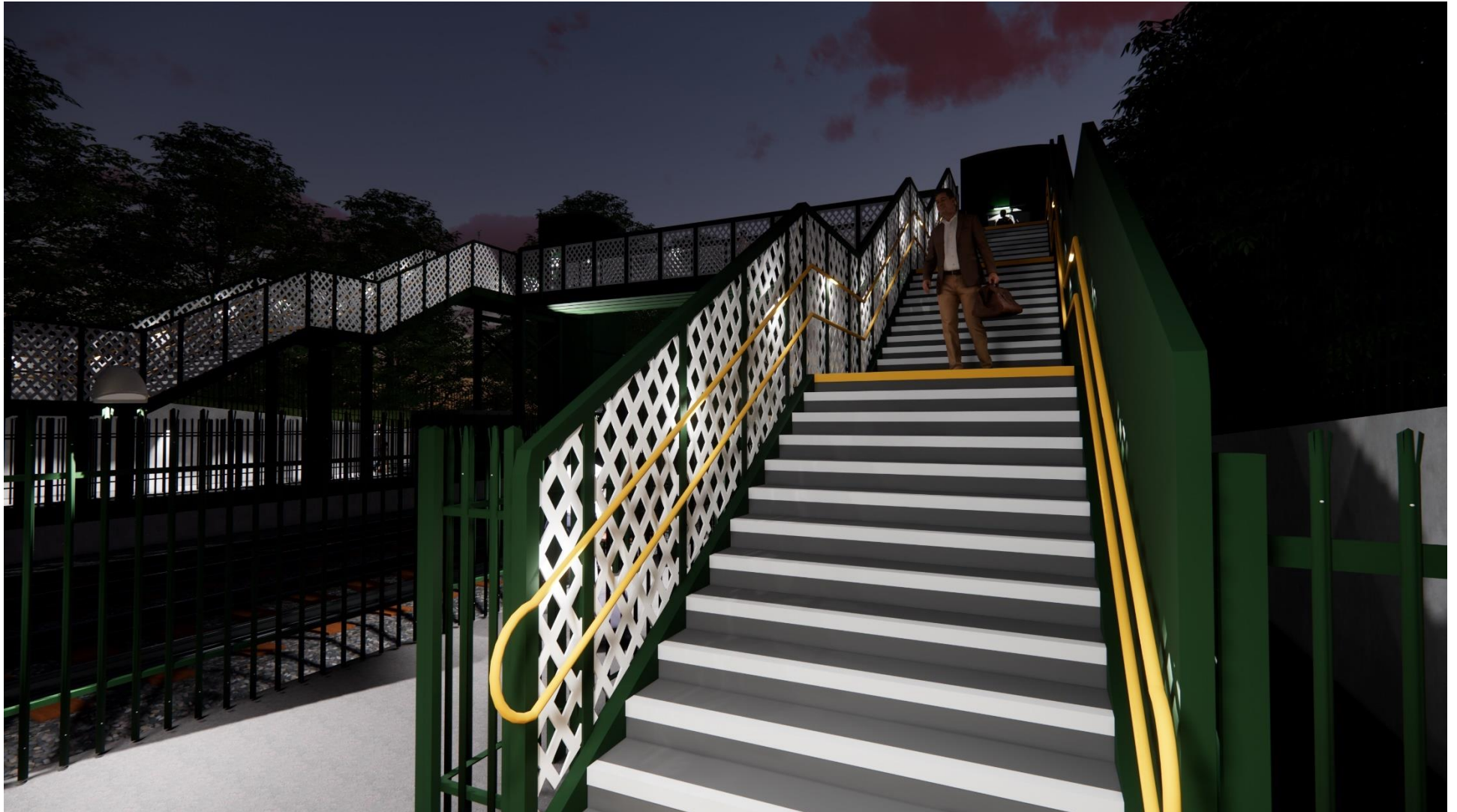
Figure A13: Down side staircase, showing the effect of handrail lighting for maintaining visibility of steps for bridge users. The solid down side parapet is also clearly visible.
