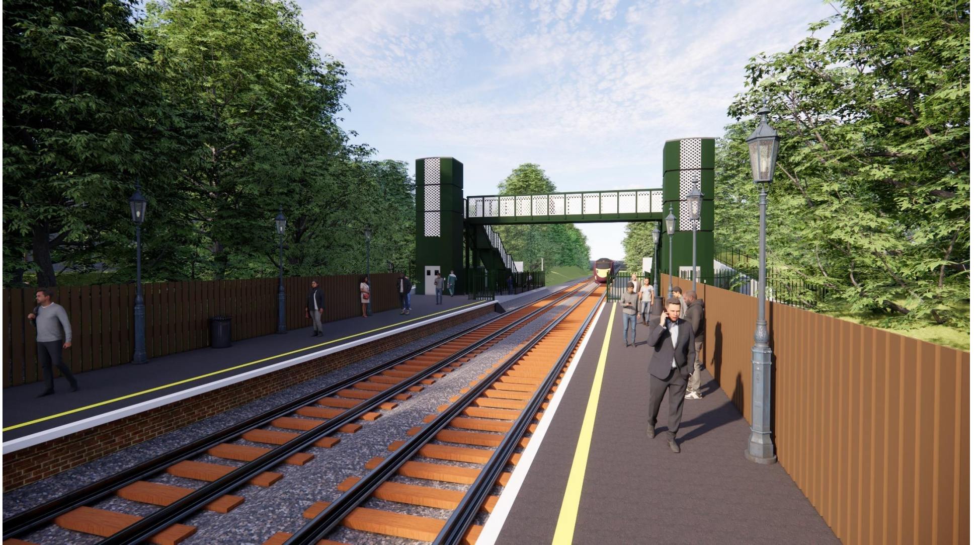
Figure A9: View of the structure from the centre of Platform 2, looking north.
