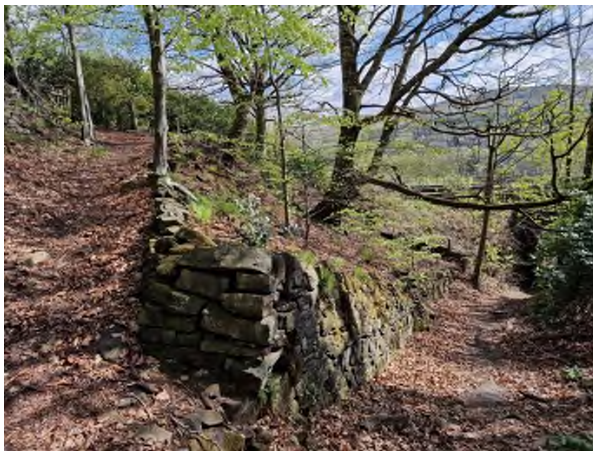
Photo 5.8f – Section of Public Footpath (looking West, uphill)
