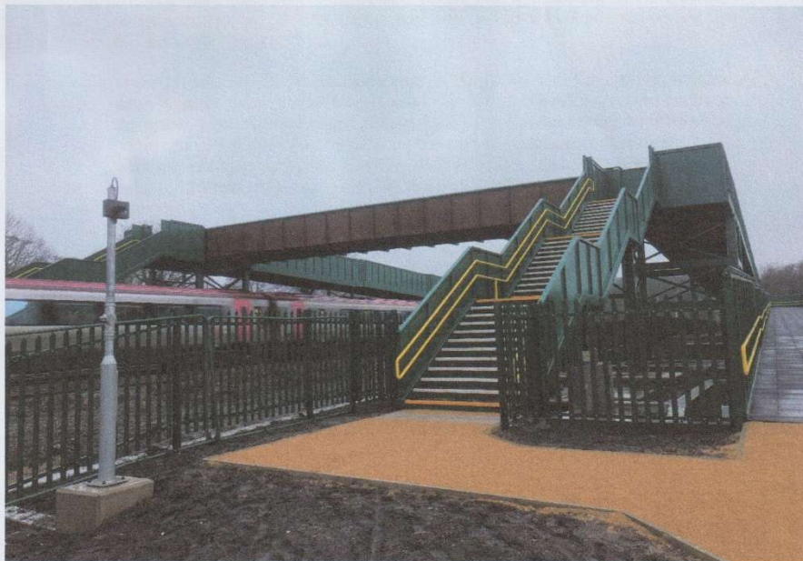
Bridleway/footbridge as completed – 30 January 2026
