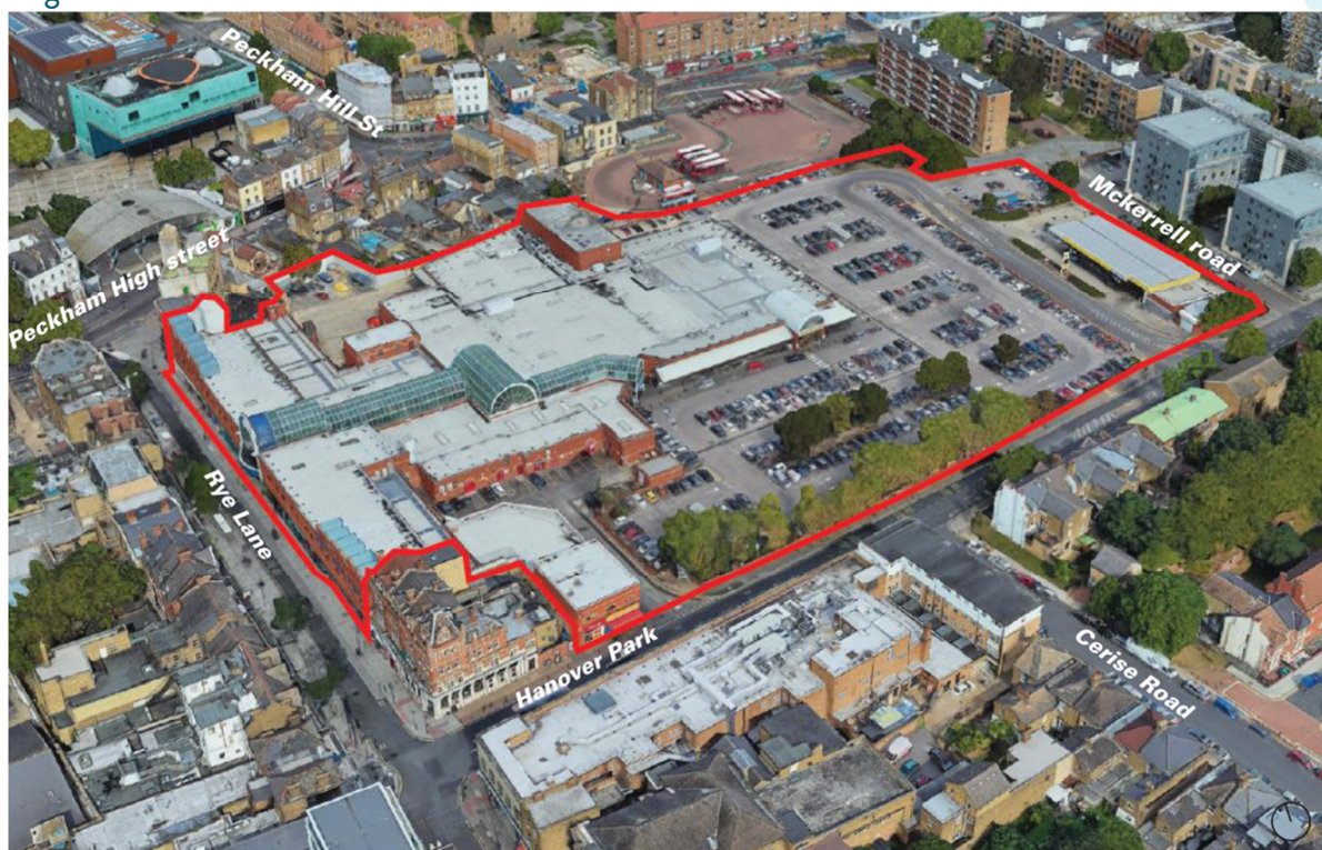
Figure 1.2– Site aerial view
