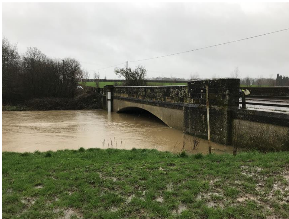
Figure 5: The bridge on Ensfield Road over the River Medway, 12:37 on 16 February 2020
