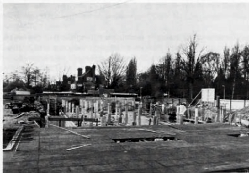
18. Foundations for the Clare Hall buildings, 1967.
