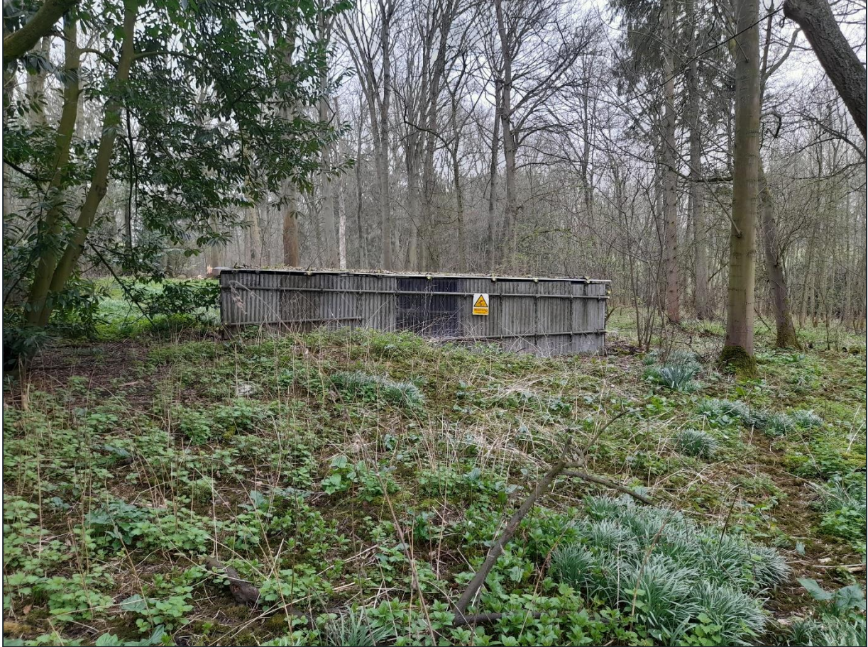
Plate 5-6-4-1 - Corrugated sheet metal encapsulating the icehouse
