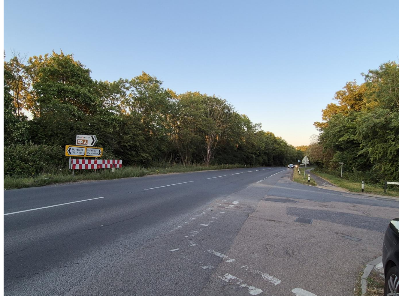
Long Road, St Neots junction, day-time photo
