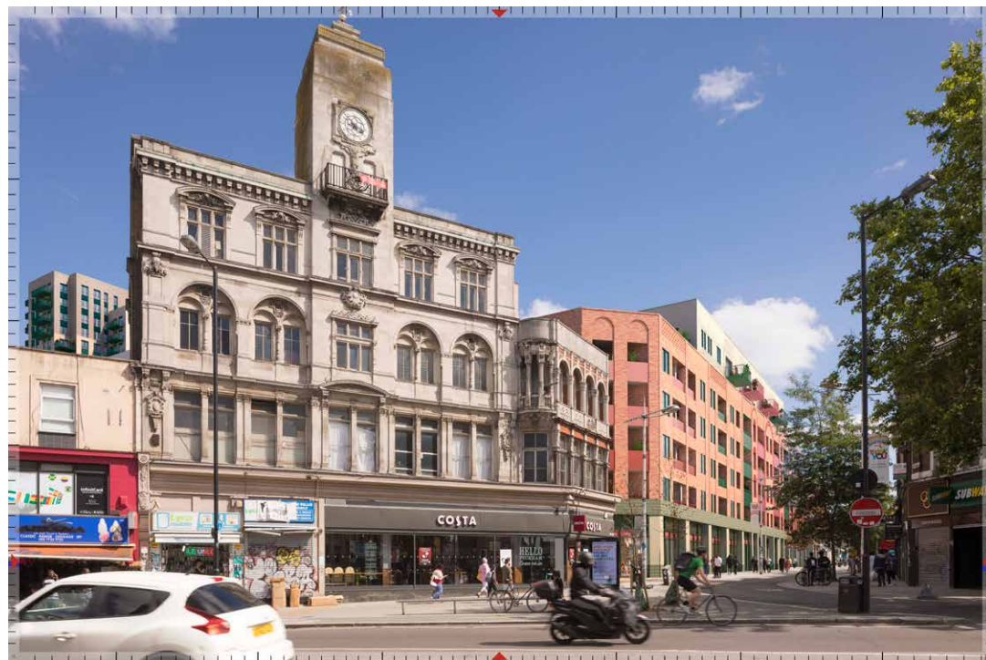
View looking south from Peckham High Street and Rye Lane junction (View 6)
