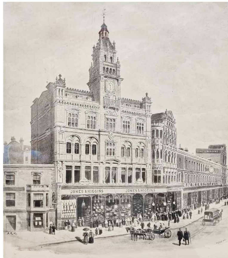
Original J&H clocktower building
