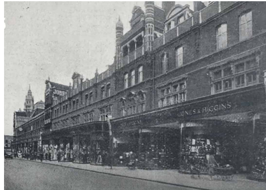
View north-east up Rye Lane at the expanded Jones and Higgins store.
