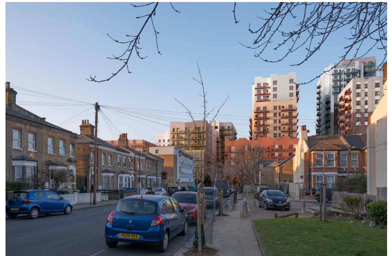
Looking north-east towards building J from Hanover Park (View 36)
