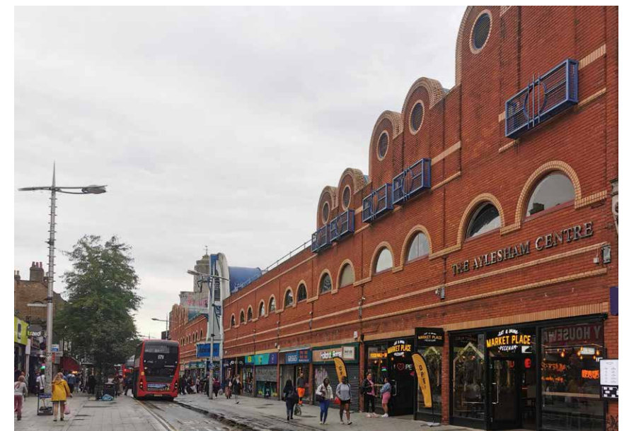
View north up Rye Lane at the existing Aylesham Centre - built 1988 after Jones and Higgins closed in 1980.
