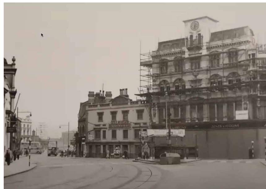
View of the Clock Tower, at the Rye Lane - Peckham High Street junction being rebuilt out of stone
