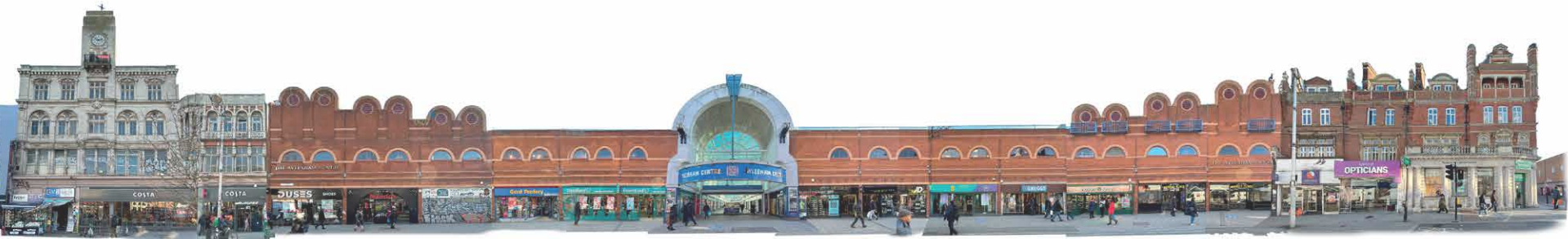
Rye Lane east elevation - ground floor commercial
