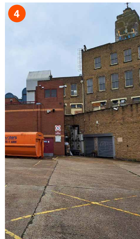
Rye Lane Service Yard
