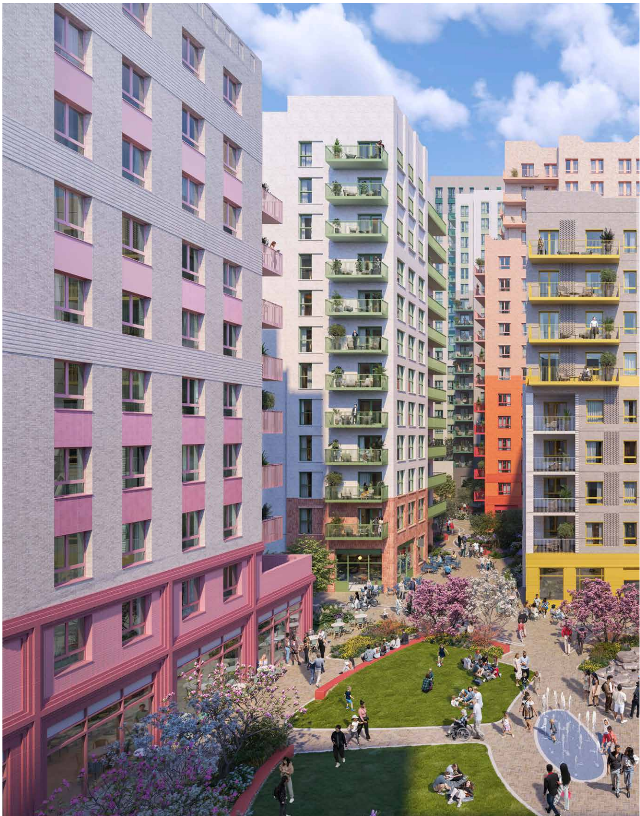
Building E facing Aylesham Gardens
