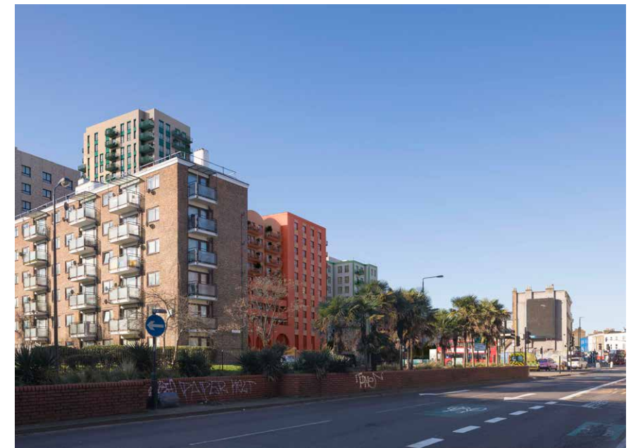
View from the junction between Peckham High Street and Marmot St (View 28)
