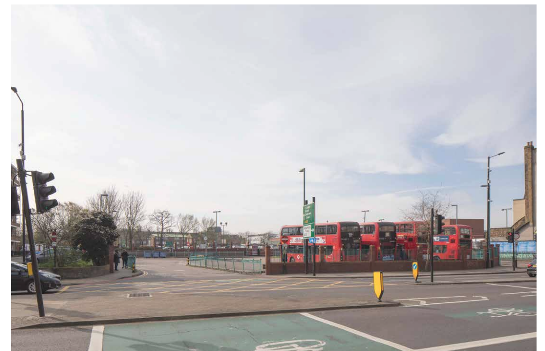
View from Peckham High Street, looking across the bus station (View 37)
