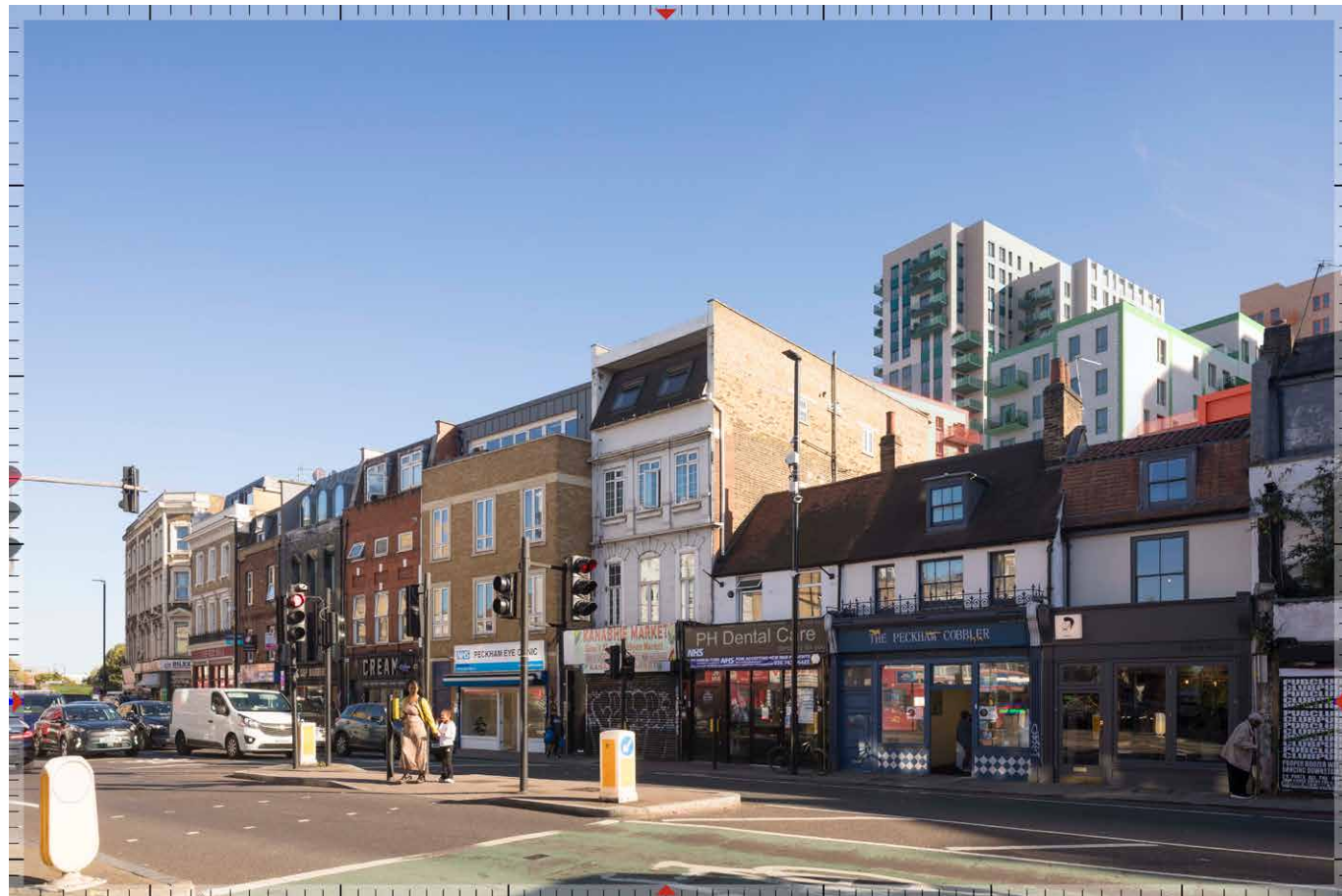
View from Peckham Hill Street / Peckham High Street, outside M. Manze (View 35)
