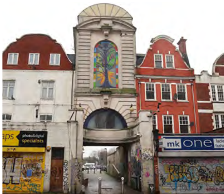
3. Existing cut through along Rye Lane
