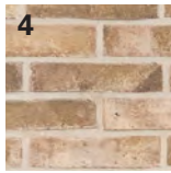
Light brown brick Light grey mortar
