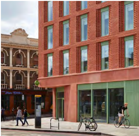
115 Camden High Street - Morris+Company
