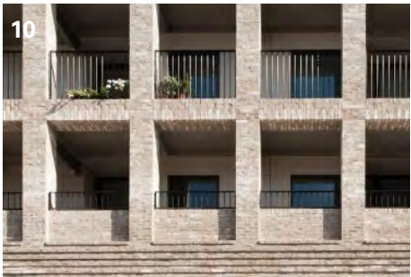
Brick pier gallery access
