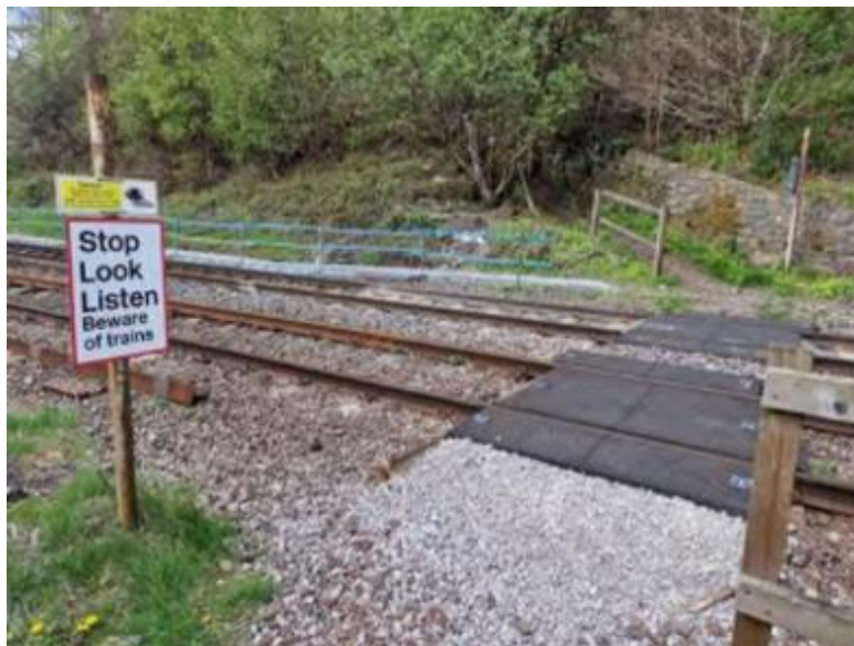
Figure 10 Moorgate Halt Existing Crossing
